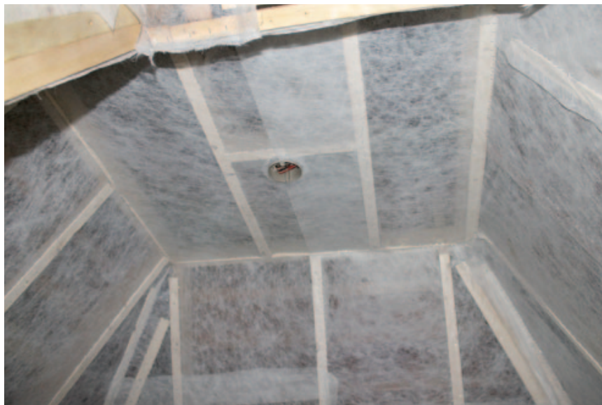
Figure 3. A skilled installer can snugly fit the netting around joists, collar ties, and other obstructions. As long as the material is tight and securely stapled, small gaps won't leak significant amounts of insulation as the cavities are blown full (right). In complex areas, like the peak of this Queen Anne tower (below), netted dense-pack can be a cost-effective alternative to spray foam.
