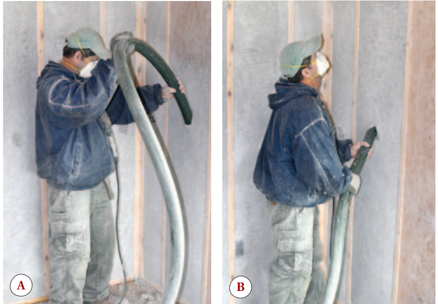
Figure 4. Wall cavities are filled first from the bottom to the midpoint of the wall (A), then from the top back to the middle (B). After a cavity is filled, the operator uses a remote control (C) to momentarily turn off the blower, then quickly inserts the hose into the next cavity before switching it on again.
