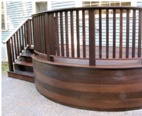
Figure 8. The numerous joints in railings make them vulnerable to water. Sealing end grain before assembly and using silicone sealant where railings meet the house help keep water out.
