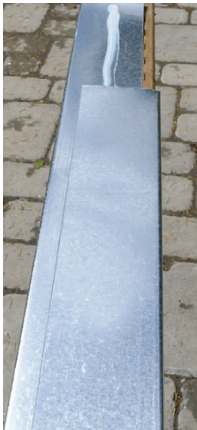
Figure 5. Two pieces of L-shaped flashing sealed with a bead of silicone protect the tops of beams.
