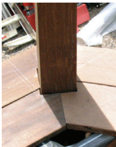
Figure 7. A bead of silicone sealant will keep water out of the joint between the railing post and the framing.
