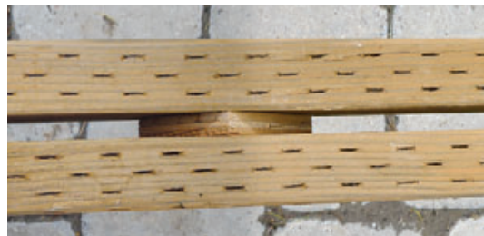
Figure 3. Spacing double joists with pieces of pressure-treated plywood allows the members to dry.
