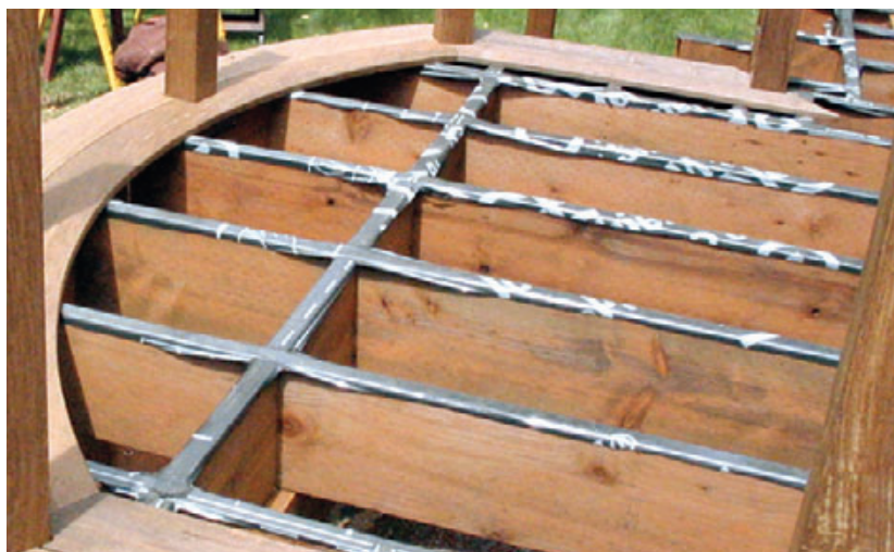
Figure 4. Flashing the tops of joists with peel-and-stick membrane protects them from water and seals penetrations from decking screws.
