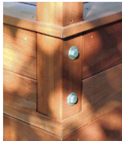
Figure 9. The end grain of decking and wood trim is coated with a preservative-sealant before assembly.
