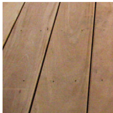
Figure 10. Deck screws loosen up as the decking shrinks. Plan to return a year or two after building the deck to retighten them.
