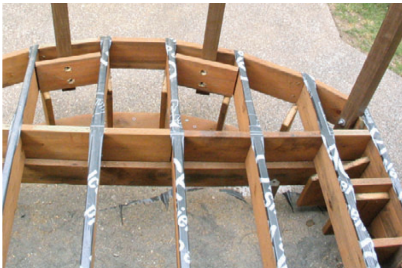
Figure 6. The complex framing used to secure railing posts makes a perfect place for water to collect.
