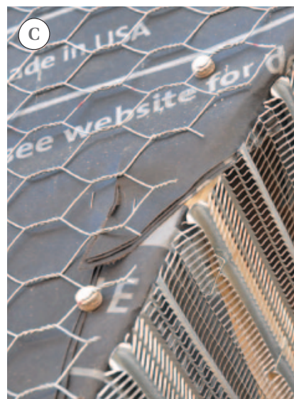
Figure 4. This wire lath (A) has been installed backward; it should be positioned so the ridges hold it away from the wall. The author advises against using staples (B) to attach lath, because the holes they make in the building paper tend to become elongated. Furring nails (C) are preferable; they have a cork washer that holds the wire off the paper and also seals around the shank.
