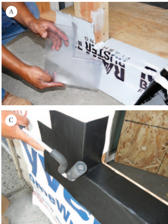
Figure 3. Prefabricated plastic corners (A) and flashing tapes and membranes (B) simplify window and door installation. Always use a roller when installing self-adhering membranes, to get rid of wrinkles (C).
