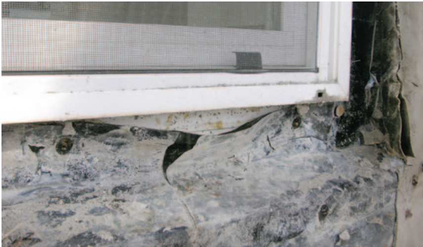
Figure 2. This window's bottom flange was taped to the sheathing (above). Trapped water caused the flashing membrane's adhesive to fail, directing even more water into the framing. Wrinkles in the membranes can also create water paths underneath stucco, as in the wide sill of this recessed window (right).
