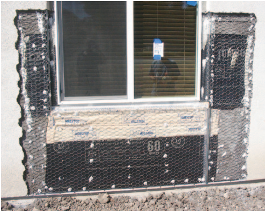
Figure 6. The open slits in the upper leg of this poorly installed weep screed (top) allowed water to soak the framing. Above, a wall has been repaired and is ready for stucco. The upper leg of the screed is behind the building paper as it should be, but there is not enough clearance to grade.
