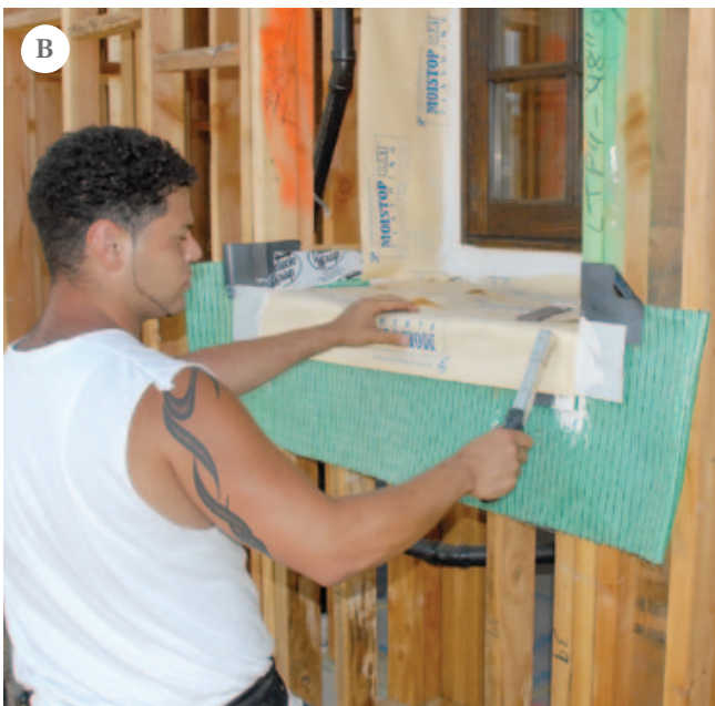
Figure 3. Prefabricated plastic corners (A) and flashing tapes and membranes (B) simplify window and door installation. Always use a roller when installing self-adhering membranes, to get rid of wrinkles (C).
