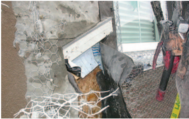
Figure 1. Shown here (above) is a shutter block that was installed on top of a piece of light-blue self-adhered flashing. Unfortunately, the building paper was then installed on top of the flashing beneath the block, which allowed water to run behind the paper and soak the framing. In the repair (right), the flashing membrane sits on top of the paper below the block.
