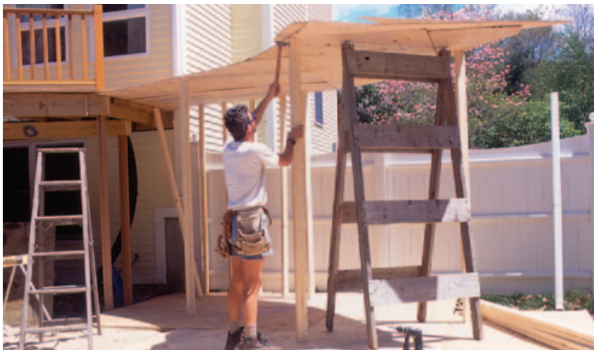
Figure 2. After scribing the stair on the plywood on the ground, the author makes a mirror image of the layout from a double layer of plywood, adding 3½ inches — a stud width — to both edges (above). He then supports the upper template on temporary posts at deck height (right).
