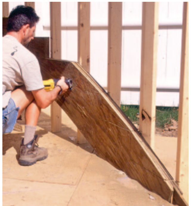
Figure 5. Plumb and level lines mark the treads and risers (left). The author makes initial cuts with a circular saw and finishes up with a recip saw to avoid overcutting the inside corners (above).
