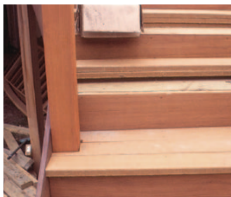
Figure 7. When stringers require intermediate support, the author uses tube forms to grade (top), then extends the wooden posts up through the framing to double as guardrail posts (above). He uses fascia material for the finished skirtboards and decking for the treads (right).
