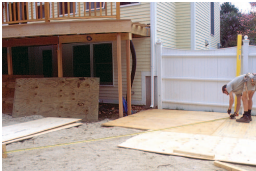
Figure 1. Swinging a tape from a wooden stake, the author lays out the inner and outer arcs of the stair at full scale on a double layer of plywood (above), then swings the walk line a foot inside the inner arc. Tread locations are marked at 10-inch-minimum intervals (right). Chalk lines snapped from the stake through the tread marks on the walk line (below) define the size and shape of the treads. The author verifies that the minimum tread width is at least 6 inches.
