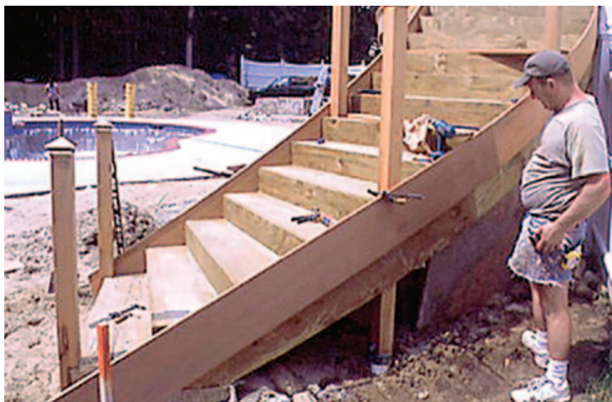
Figure 7. When stringers require intermediate support, the author uses tube forms to grade (top), then extends the wooden posts up through the framing to double as guardrail posts (above). He uses fascia material for the finished skirtboards and decking for the treads (right).
