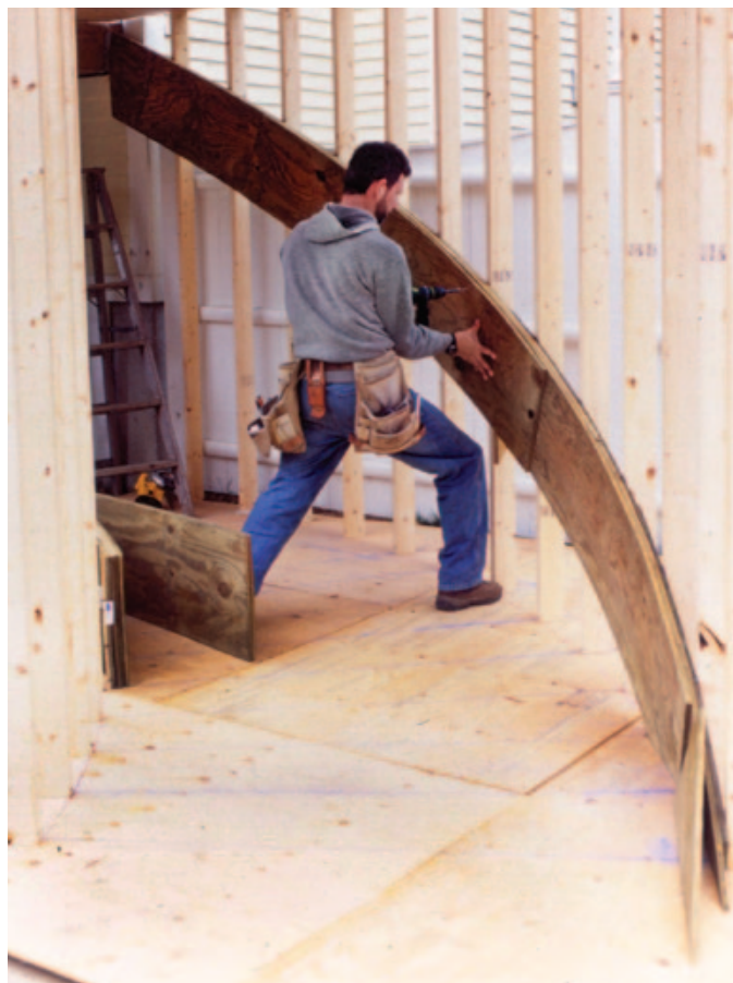
Figure 4. Using a story pole, the author marks the tread elevations on the bending frame (above). He then installs the stringer laminations, aligning the top edges with the marks and gluing and screwing them together (right).
