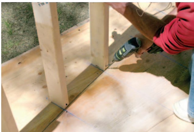
Figure 3. Straight, wane-free studs screwed to the plywood templates behind each riser line provide a bending form (above). Once built, the form is plumbed and securely braced (right).
