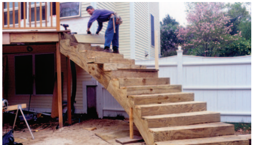
Figure 6. The risers are made from two layers of \frac{3}{4} -inch plywood lapped so as to support the front and back edges of the 2-by structural treads (illustration). The author starts installation at the bottom (top photo) and works up the stair as high as he can until he has to remove the bending frame (above).
