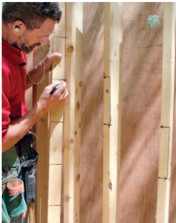
Figure 4. Using a story pole, the author marks the tread elevations on the bending frame (above). He then installs the stringer laminations, aligning the top edges with the marks and gluing and screwing them together (right).
