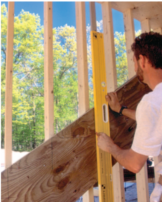
Figure 5. Plumb and level lines mark the treads and risers (left). The author makes initial cuts with a circular saw and finishes up with a recip saw to avoid overcutting the inside corners (above).
