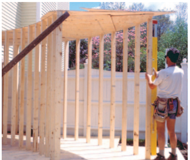
Figure 2. After scribing the stair on the plywood on the ground, the author makes a mirror image of the layout from a double layer of plywood, adding 3½ inches — a stud width — to both edges (above). He then supports the upper template on temporary posts at deck height (right).
