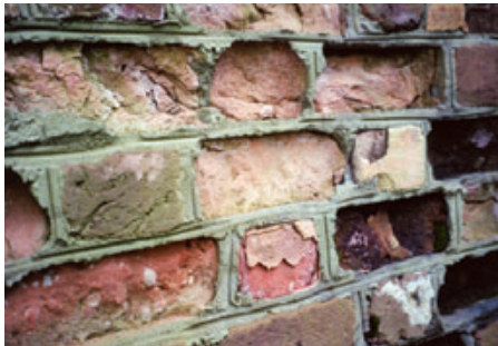
This garden wall was built with salvaged fill bricks. Over time, the porous bricks absorbed water, which eventually froze and expanded, causing the face of the bricks to spall.
