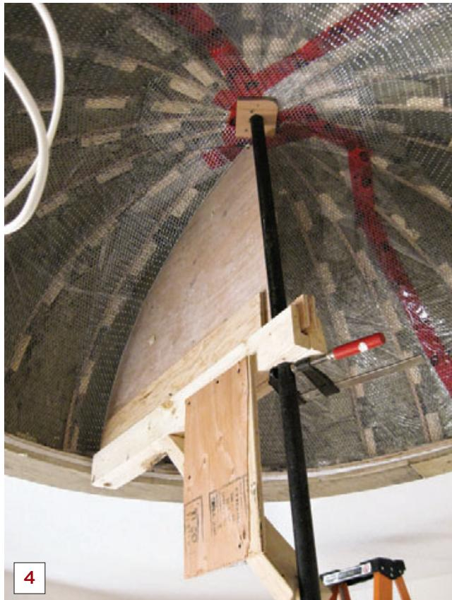
screed to strike it off at a uniform thickness, working in sections because the material set up quickly. Since the plywood base ring was slightly smaller than the base of the dome itself — forming a ledge that would later accommodate a string of rope lights — we had to disassemble and remove the screed between coats. Then we used a belt sander to remove a small amount of material from the leading edge to account for the thickness of the next coat.
