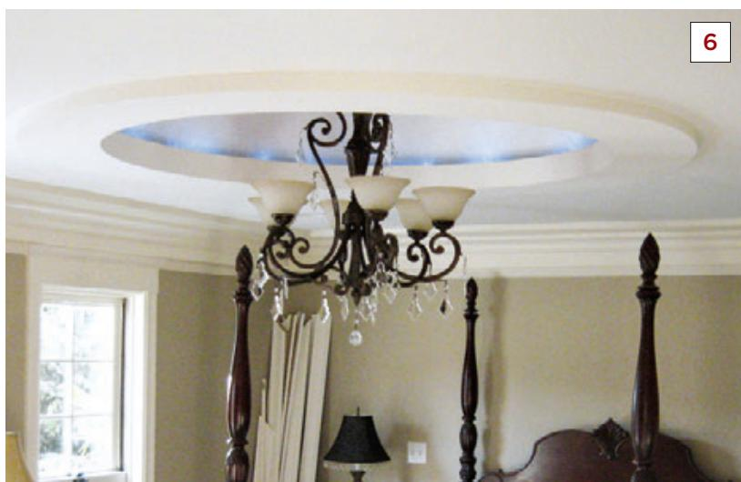
edges of the plywood ring and mudded them. The exposed face of the ring received a skim coat of mud at the same time. Finally, we installed a ceiling medallion at the peak (5) and wired the rope lights and hanging light fixture (6).
