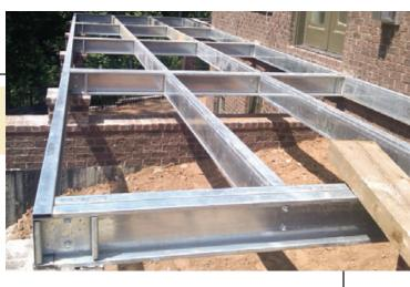
bled with self-tapping screws or 1/2-inch bolts, or they can be welded.
