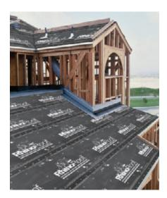
a slip-resistant texture and is easily chalked, says the company. It's suitable for use only with asphalt shingles. The manufacturer declined to provide pricing.
