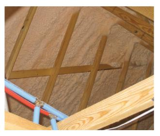
Fireproof Foam. *GacoFireStop* is the first opencell foam approved for use in attics and crawlspaces with no additional ignition barrier. According to the maker, the insulation has passed the AC 377 Appendix X test for flammability twice: shaved, and with the skin on. It's NFPA-approved for 12-inch-maximum wall thicknesses and 16-inch-maximum ceilings. Installation costs for an R-19 wall assembly average \$3 per square foot, and for an R-38 ceiling about \$6 per square foot.
