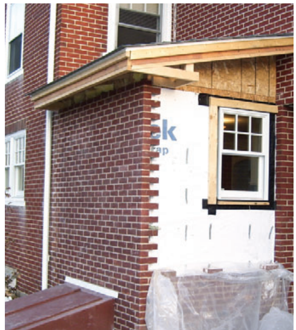
Figure 6. The crew left a section of sheathing off the addition so they could more easily remove the brick from inside (top). Where the addition met the original house, the new and existing bricks were toothed together beside a downspout to help hide the transition (above).
