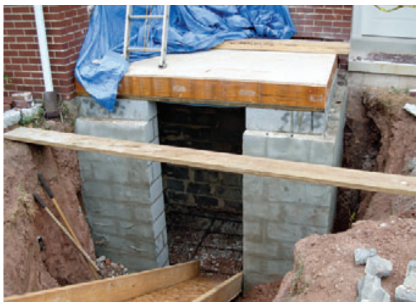
Figure 3. The block foundation of the small addition includes a shelf for the new brick veneer. After the deck was framed and the new masonry walls stabilized, a new precast bulkhead was craned into place.
