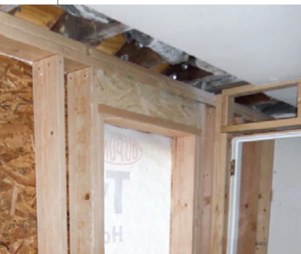
Figure 10. Birdsmouths were cut into the rafters to accommodate the new 2x6 wall framed on top of the Parallam (left). The face of the sheathing is 1½ inches behind the back of the stone to allow for drainage (above).
