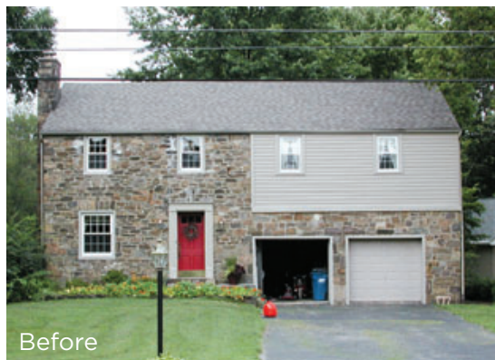
Figure 7. An earlier master-bedroom addition above the garage was clad with vinyl siding (left); the new owners wanted to replace the vinyl with local stone that matched the rest of the front facade (above).
