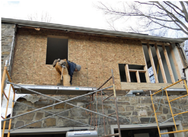
Figure 10. Birdsmouths were cut into the rafters to accommodate the new 2x6 wall framed on top of the Parallam (left). The face of the sheathing is 1½ inches behind the back of the stone to allow for drainage (above).
