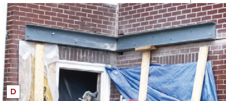
Figure 4. Working off the 6-foot-by-8-foot deck of the addition, the crew first kerfed the mortar joints to receive the steel angle (A) and made a hole to allow the 14-foot channel to pass inside at the second-floor level (B). The longer channel was installed first and bolted into place (C), then the shorter channel (D). The right-angle joint at the intersection of the steel channels was later welded.
