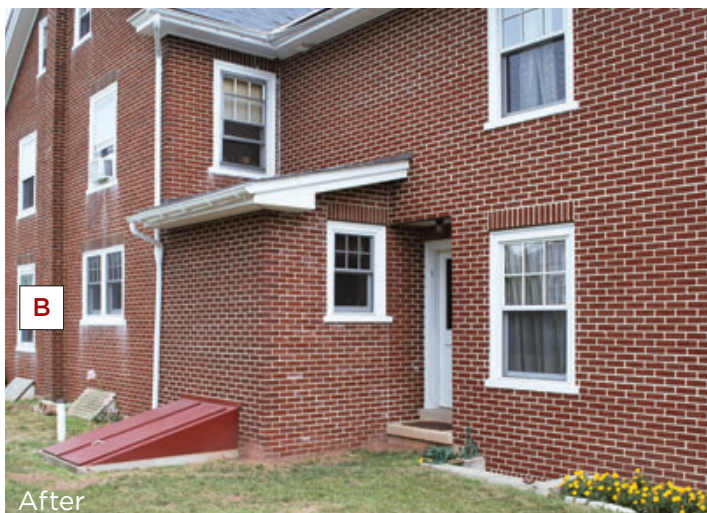
Figure 1. A 48-square-foot addition on the back corner of this brick home created a larger rectangular space for the kitchen. The project required removing the first-story structural brick wall in the inside corner and supporting the second story with steel beams. Note the boxed-out column at the right rear of the new refrigerator (D), which encloses a lally column positioned where the original exterior wall used to be.
