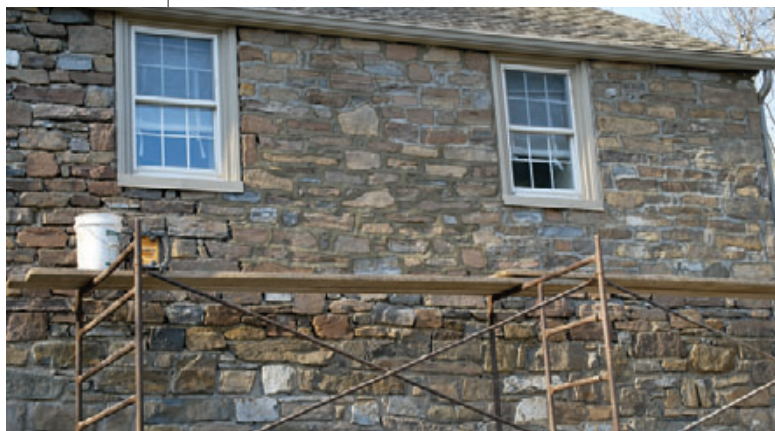
Figure 11. The original windows were reinstalled on plywood extension jambs set into the new frame wall (top). The new locally quarried stones should weather to more closely match the original (above).
