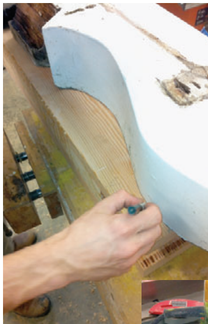
Figure 1. The 2x10 fir laminations of the partial replacement posts are offset to create a slot for joining to the original post sections (far left). After scribing the original column patterns (left) and cutting them out on a band saw, the author created a matching tongue profile with a router (below).
