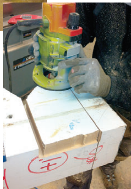
Figure 1. The 2x10 fir laminations of the partial replacement posts are offset to create a slot for joining to the original post sections (far left). After scribing the original column patterns (left) and cutting them out on a band saw, the author created a matching tongue profile with a router (below).
