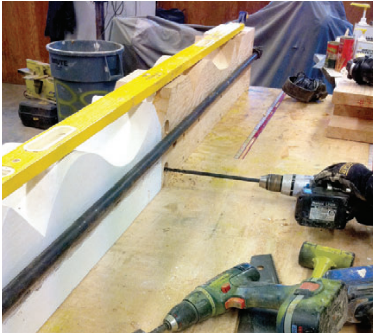
Figure 2. The new and old column sections were joined together with galvanized through-bolts and epoxy (above). Once the columns were reassembled, a worker straightened them with a large-capacity beam saw (right).
