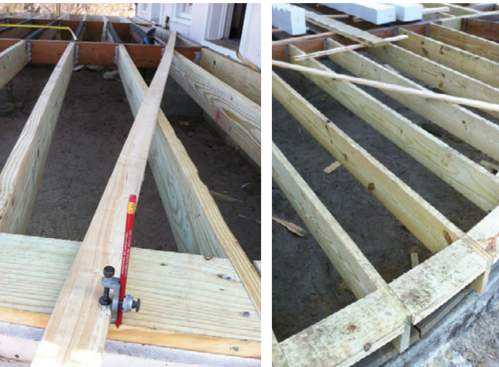
Figure 3. The author replaced the rotted joists with treated framing, then used a trammel arm (left) to scribe the deck's radius onto blocking installed on the flat around the perimeter of the deck (right).
