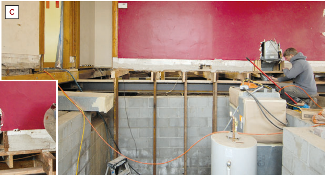
Figure 4. LVL ledgers attached to the exterior wall studs with structural screws (A) provided a means of support as the sill was removed and the steel beam maneuvered into place (B). At the center bearing wall, the crew had to work around the temporary supports under the short joist remnants as the steel was inserted (C). To make this process easier, the beam was fabricated in sections designed to be bolted together on site (D).
