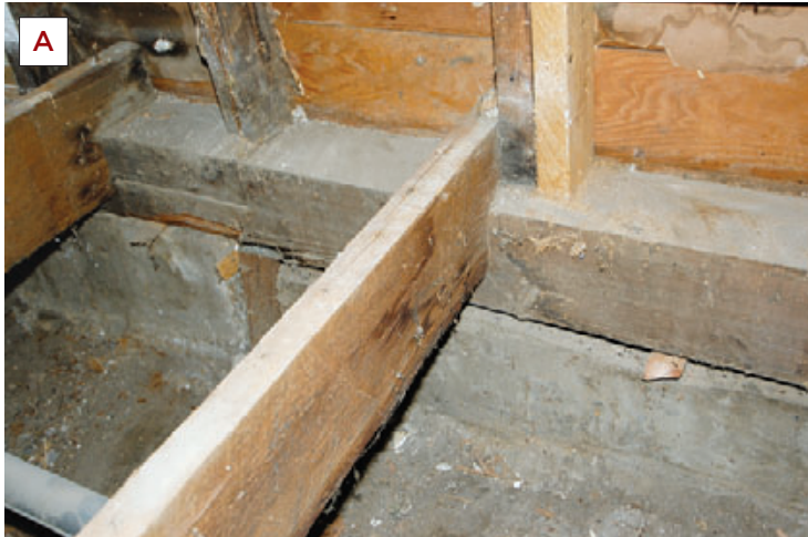
Figure 2. The exterior walls were balloon-framed, with the joists notched into the original sill; here it would be easy to pull the joists without disturbing the walls (A). At the center girder, however, the crew had to provide shoring with short blocks set on plates (B) so that the first-story bearing would be supported as the joists were cut away (C).
