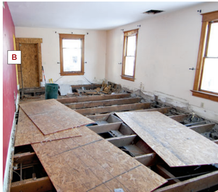
Figure 1. The author began by removing the original flooring (above) to expose the foundation and floor framing (right). Ductwork, wiring, bathroom fixtures, and plumbing also had to be pulled.
