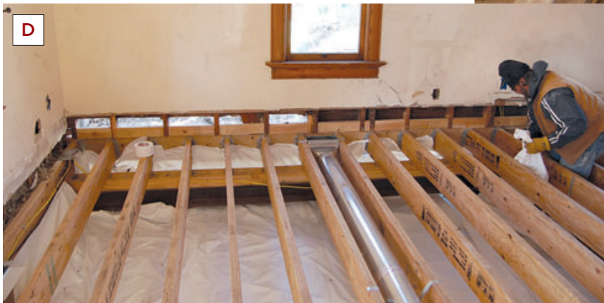
Figure 5. Working a wall section at a time, the crew cut the studs off and extended them to the new girder under the bearing wall (A). Along the outside walls, a double rim was installed from outside at the same elevation as the original sill (B); upside-down joist hangers help transfer roof loads to the new steel beam (C). A heavy vapor retarder (D) will help keep the crawlspace dry.
