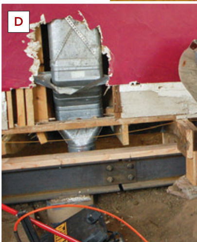
Figure 4. LVL ledgers attached to the exterior wall studs with structural screws (A) provided a means of support as the sill was removed and the steel beam maneuvered into place (B). At the center bearing wall, the crew had to work around the temporary supports under the short joist remnants as the steel was inserted (C). To make this process easier, the beam was fabricated in sections designed to be bolted together on site (D).
