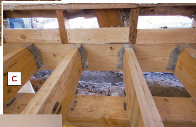
Figure 5. Working a wall section at a time, the crew cut the studs off and extended them to the new girder under the bearing wall (A). Along the outside walls, a double rim was installed from outside at the same elevation as the original sill (B); upside-down joist hangers help transfer roof loads to the new steel beam (C). A heavy vapor retarder (D) will help keep the crawlspace dry.
