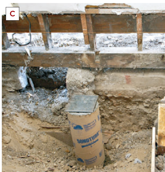
Figure 3. Around the perimeter of the building, a specialty subcontractor installed helical piers as close to the foundation walls as practical (A). Given the region's expansive clay soils, the lead helix was driven to a depth of around 30 feet. The pier contractor then cut the tops of the extension shafts to a uniform height and welded on a steel plate fitted with rebar dowels (B). Each pier was topped with a steel-reinforced concrete pier; a steel bearing plate was embedded in the wet concrete at exact finish height (C).
