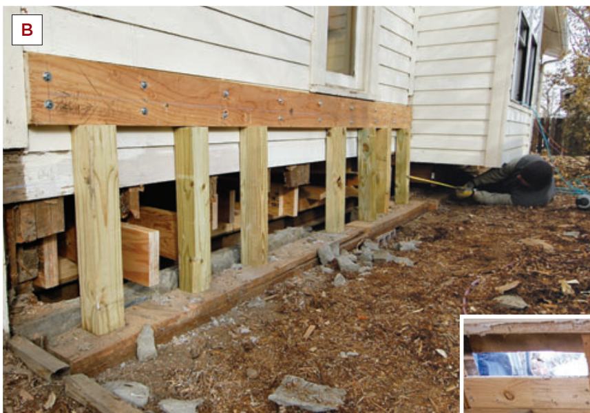
Figure 5. Working a wall section at a time, the crew cut the studs off and extended them to the new girder under the bearing wall (A). Along the outside walls, a double rim was installed from outside at the same elevation as the original sill (B); upside-down joist hangers help transfer roof loads to the new steel beam (C). A heavy vapor retarder (D) will help keep the crawlspace dry.
