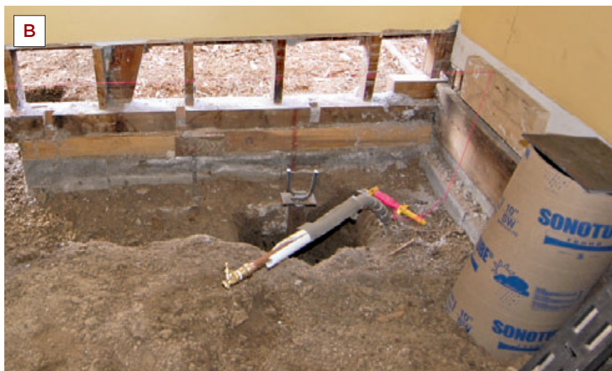
Figure 3. Around the perimeter of the building, a specialty subcontractor installed helical piers as close to the foundation walls as practical (A). Given the region's expansive clay soils, the lead helix was driven to a depth of around 30 feet. The pier contractor then cut the tops of the extension shafts to a uniform height and welded on a steel plate fitted with rebar dowels (B). Each pier was topped with a steel-reinforced concrete pier; a steel bearing plate was embedded in the wet concrete at exact finish height (C).
