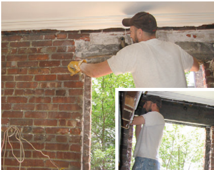
Figure 2. After removing the door and window, a carpenter begins chipping away enough of the inner wythe of brickwork over the openings to install a section of C10x20 steel channel, the first half of the header assembly (left). The outer wythe of brick will remain in place during the installation to maintain the wall's structural integrity (below).
