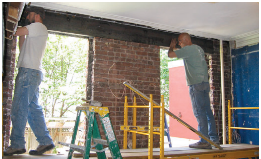
Figure 2. After removing the door and window, a carpenter begins chipping away enough of the inner wythe of brickwork over the openings to install a section of C10x20 steel channel, the first half of the header assembly (left). The outer wythe of brick will remain in place during the installation to maintain the wall's structural integrity (below).
