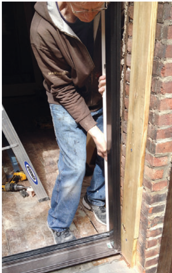
Figure 5. Finally, the old wall is capped with a new concrete sill to create a flat and level opening for the new door (above). Treated 5/4 bucks and the door itself are installed by a subcontractor (left).
