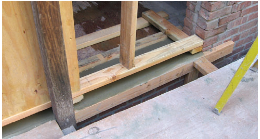
Figure 5. Finally, the old wall is capped with a new concrete sill to create a flat and level opening for the new door (above). Treated 5/4 bucks and the door itself are installed by a subcontractor (left).
