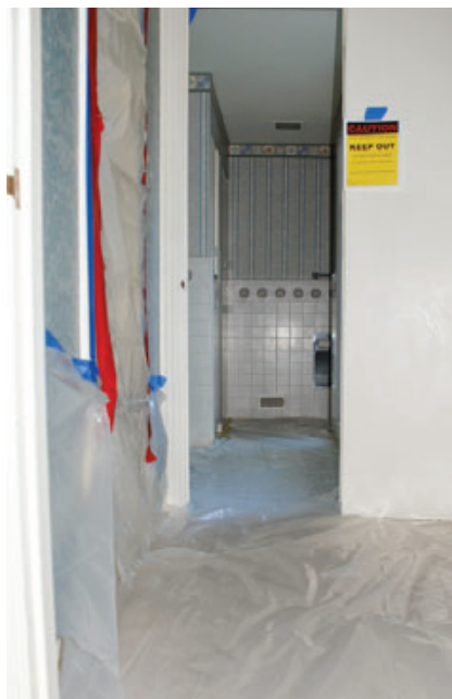
Before performing the demolition phase of this bathroom remodel, the author covered the floors, doors, and adjacent appliances with plastic, then posted his warning signs. Because he completed the RRP and cleanup phase of the project immediately after demolition, complying with the lead rule cost only about $35 in materials and required two hours of labor.
