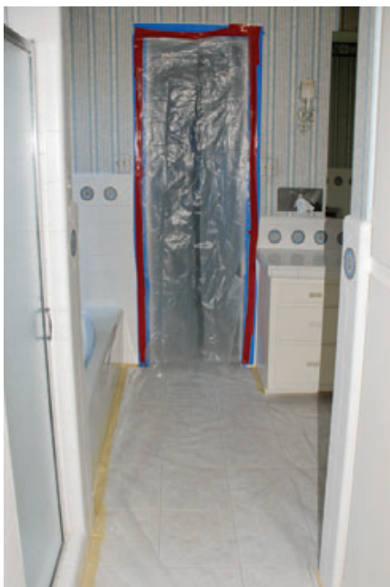
Before performing the demolition phase of this bathroom remodel, the author covered the floors, doors, and adjacent appliances with plastic, then posted his warning signs. Because he completed the RRP and cleanup phase of the project immediately after demolition, complying with the lead rule cost only about $35 in materials and required two hours of labor.
