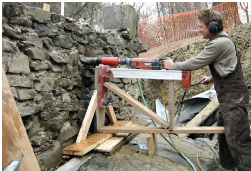
Figure 5. An improvised stand supports the coring drill used to bore 3-inch-diameter holes for the wall tiebacks. To provide an aiming point, a length of white closet rod — visible at top left — was inserted in the previously drilled vertical holes extending from top to bottom of the wall.
