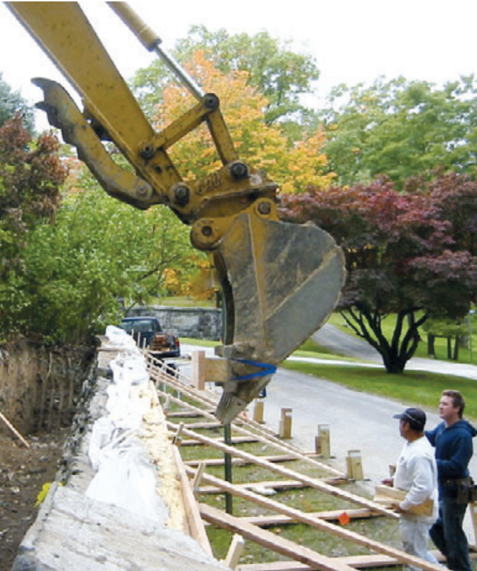
Figure 3. A heavy wood block strapped to the excavator's bucket (left) distributed the pressure across a 4-foot section of shoring as the wall was eased upward. Though relatively little lifting force was needed, only a large machine could supply the necessary reach across the excavation. The wall's battered configuration — wider at bottom than top — increased its stability in the fully upright position (above).
