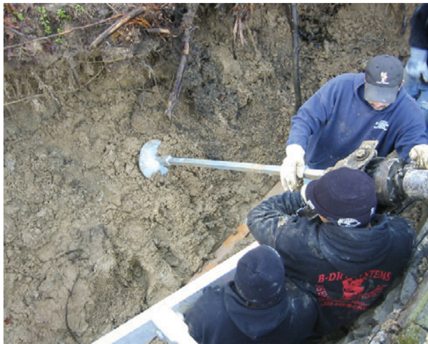
Figure 4. Helical soil anchors furnished tieback points for fixing the reinforced wall to the hillside. The anchor sub was familiar with retaining-wall design and recommended an appropriate depth and spacing for the anchors.
