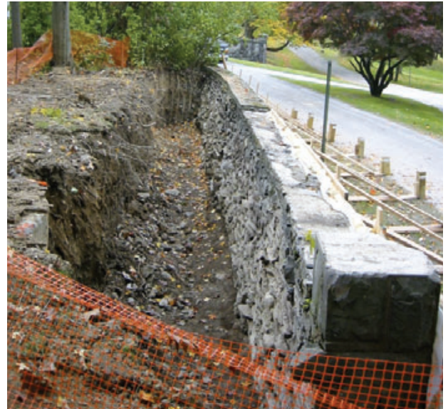
Figure 3. A heavy wood block strapped to the excavator's bucket (left) distributed the pressure across a 4-foot section of shoring as the wall was eased upward. Though relatively little lifting force was needed, only a large machine could supply the necessary reach across the excavation. The wall's battered configuration — wider at bottom than top — increased its stability in the fully upright position (above).
