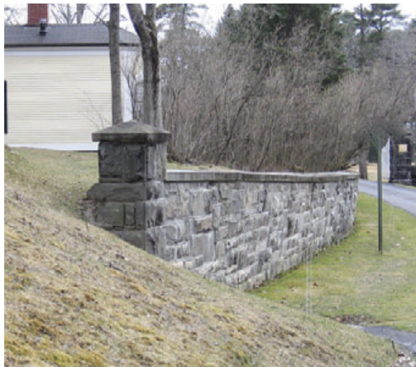
Figure 8. The restored section of the wall stands perfectly straight. To save the mature plantings visible at rear, repairs were limited to the most severely affected section; parts of the original wall remain several inches out of plumb.
