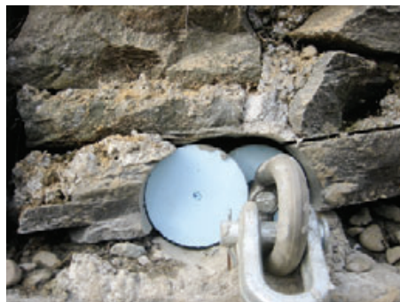
Figure 6. Strands of epoxy-coated rebar pin the repositioned upper wall to the undisturbed portion below grade (above left). The protruding ends visible here were later cut off flush with the top of the wall. The clevis removed from the bottom of the turnbuckle forms a strong mechanical connection with the rebar (above). A foam plug prevented grout from leaking out of the 3-inch-diameter horizontal holes (left).
