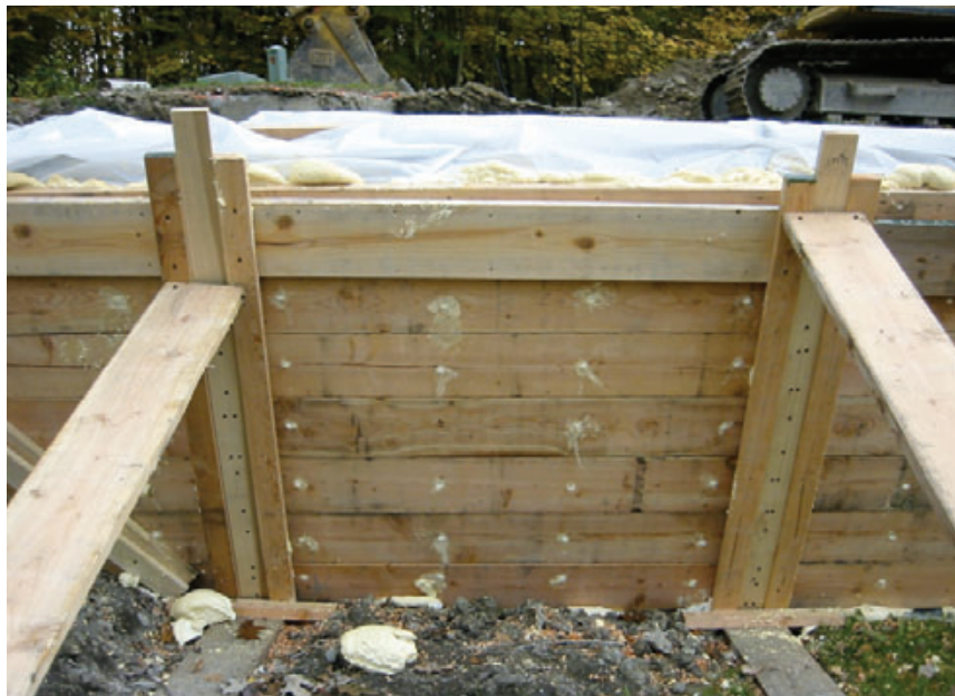
Figure 2. Closed-cell foam injected between the uneven stone wall and the shoring planks ensured consistent contact, eliminating areas of localized stress that could have caused the wall to fracture when straightened. A 4-mil poly slip sheet kept the foam from bonding to the stone.
