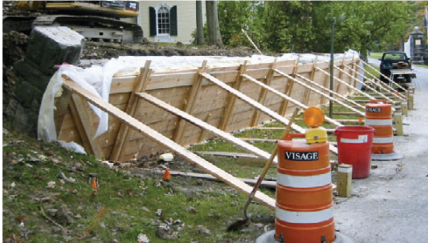
Figure 1. A system of horizontal kickers and diagonal braces bearing against 6x6 posts driven deep into the soil — one of which is visible just to the right of the traffic beacon — held the wall in position during excavation of the poorly drained original backfill.
