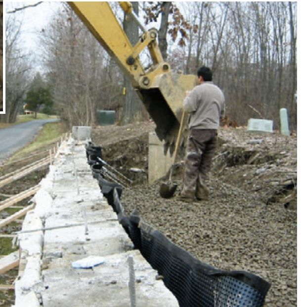
Figure 7. Once the grouted wall pins and hardware had been mechanically fastened to the exposed ends of the helical soil anchors (left), the inner face of the wall was covered with a dimpled drainage mat and the excavation was filled with stone (below).
