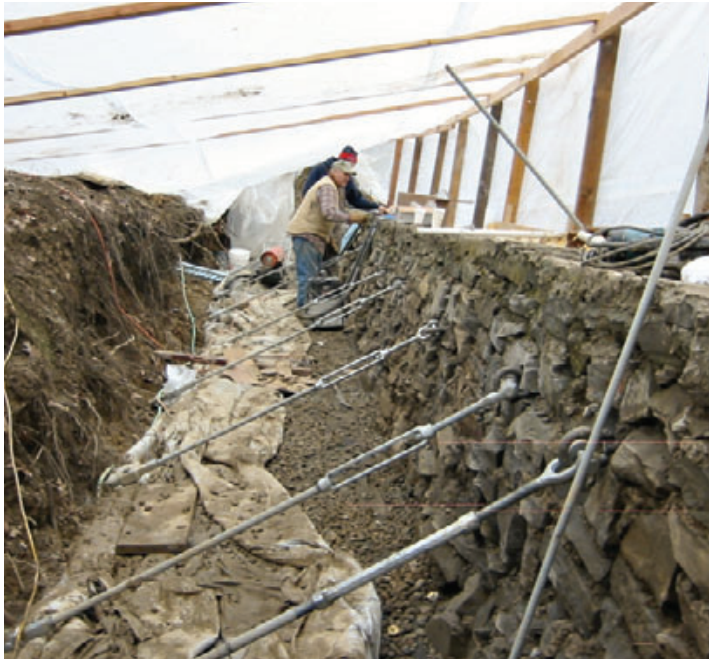
Figure 7. Once the grouted wall pins and hardware had been mechanically fastened to the exposed ends of the helical soil anchors (left), the inner face of the wall was covered with a dimpled drainage mat and the excavation was filled with stone (below).
