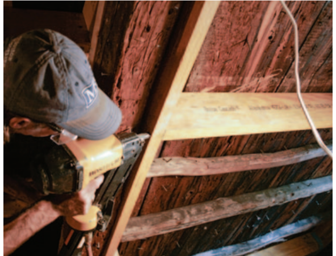
Figure 3. Bottle jacks and scraps of blocking were used to press the new LVL purlins against the roof boards (above left). A level cut at the base of each LVL sister sits flat against the existing timber plate. Working down the roof one rafter bay at a time, the crew temporarily secured each new purlin with a single nail at each end (above) before fastening the assembly permanently with joist hangers (left).
