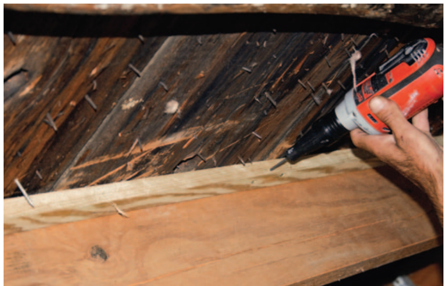
Figure 4. A 1½-inch by 1½-inch nailer fastened alternately to the purlins and the roof boards stiffens the assembly against racking without penetrating the existing roof shingles.
