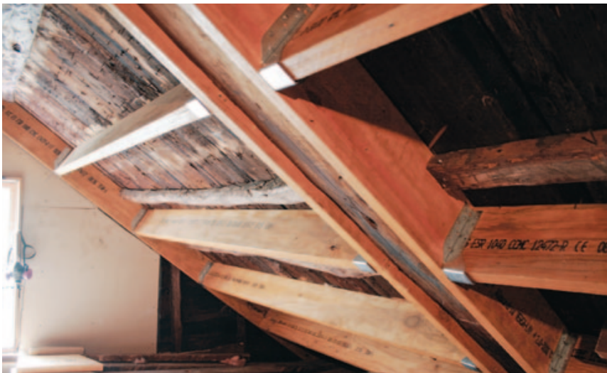
Figure 3. Bottle jacks and scraps of blocking were used to press the new LVL purlins against the roof boards (above left). A level cut at the base of each LVL sister sits flat against the existing timber plate. Working down the roof one rafter bay at a time, the crew temporarily secured each new purlin with a single nail at each end (above) before fastening the assembly permanently with joist hangers (left).
