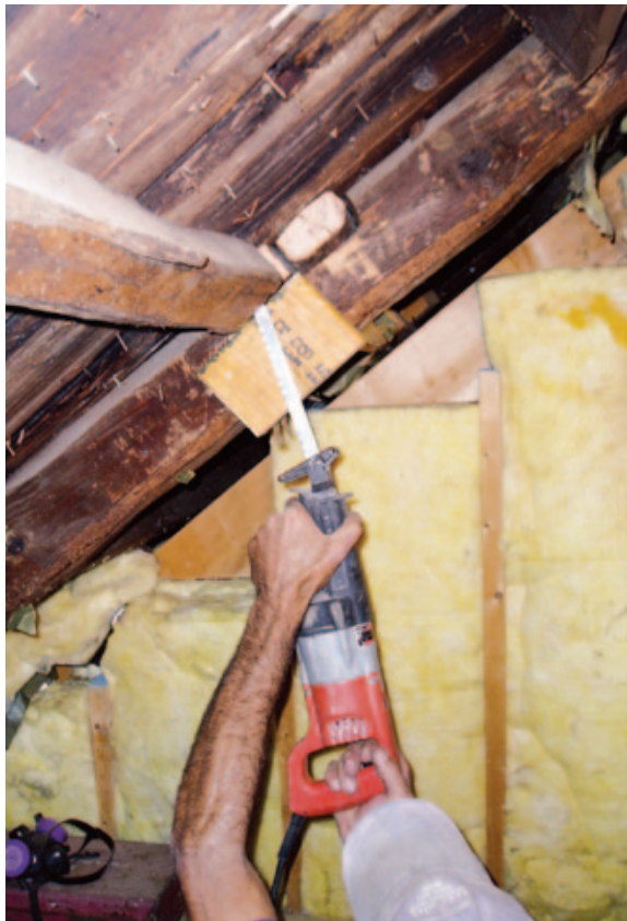
Figure 2. The original undersized purlins were small-dimensioned pieces of timber hewn flat on two sides, with some of the bark left on. Their ends were carefully cut free of the rafters, creating space to insert LVL sisters.
