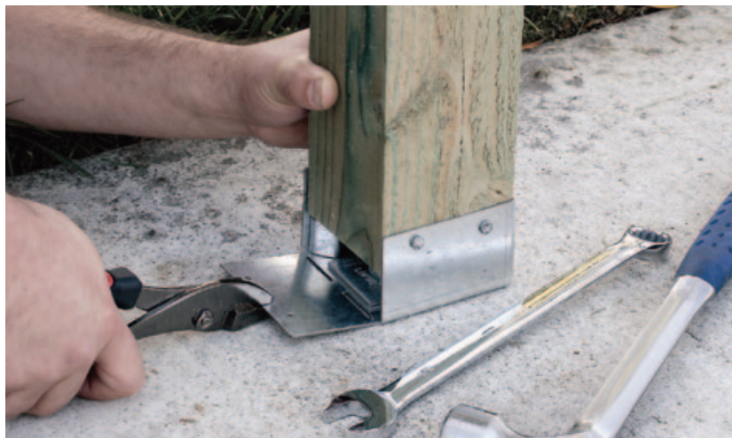
Figure 1. Most post bases fasten to a bolt that's cast or epoxied into the concrete footing. Once the post is located and the nut tightened, the base is nailed to the post.
