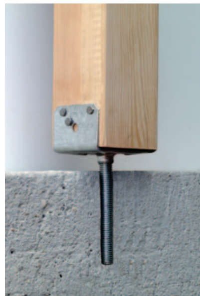
Figure 2. The height on some post bases can be adjusted with a threaded rod that's cast or epoxied into the footing.
