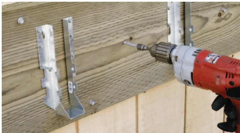
Figure 6. Far faster to install than lag screws or through-bolts, structural screws can be a great alternative for attaching ledgers.
