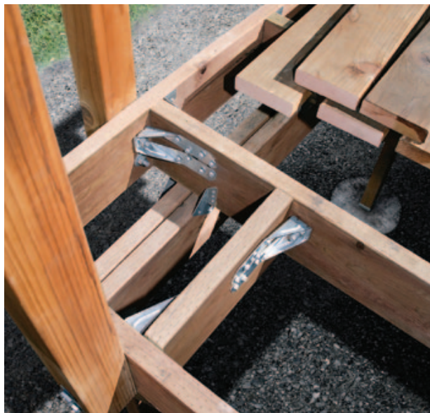
Figure 11. Railing posts generate tremendous leverage, and lateral attachment anchors can help transfer that force to the floor framing safely.
