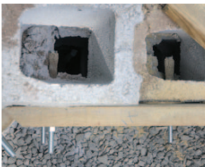
Figure 7. Epoxy anchors and bolts secure the ledger to the retaining wall.
