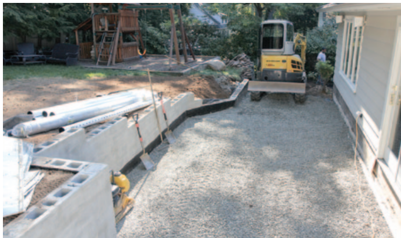
Figure 6. PVC pipe and crushed stone drain the wall. The ground below the deck was graded toward the wall, and then covered with crushed stone.
