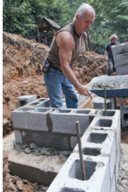
Figure 4. A mason fills the rebar-containing cells in the concrete-block retaining wall with grout.
