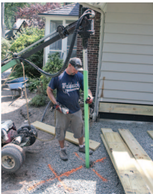
Figure 8. Galvanized steel helical-pile footings were driven to support a drop beam at the stairs.
