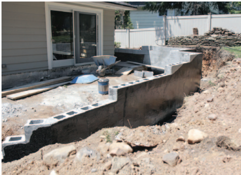
Figure 5. Portland-cement plaster and a coat of tar makes the wall water-resistant and prepares it for stone veneer.
