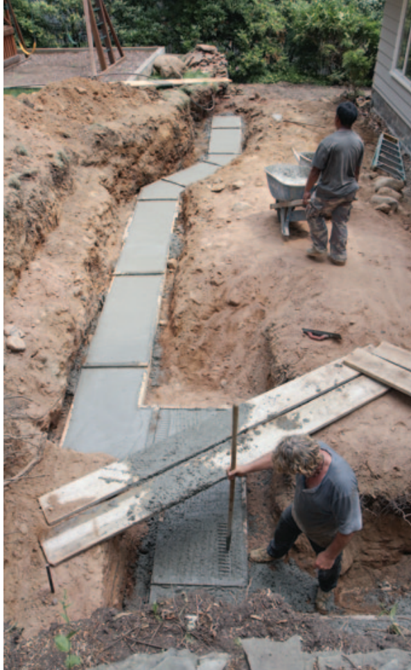
Figure 3. A concrete footing — like what you'd use for a basement wall — was poured to support the new retaining wall.
