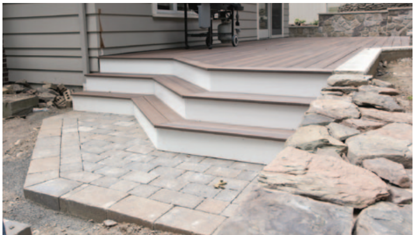
Figure 11. Concrete pavers provide a stair landing and a path to the deck.
