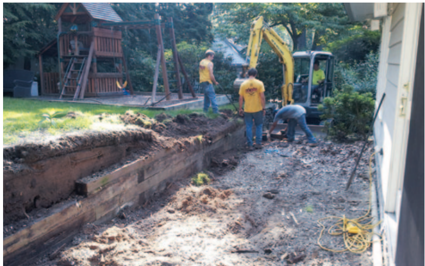
Figure 1. Problems with this job included a sunken backyard, poor drainage, and an old retaining wall that had to go.
