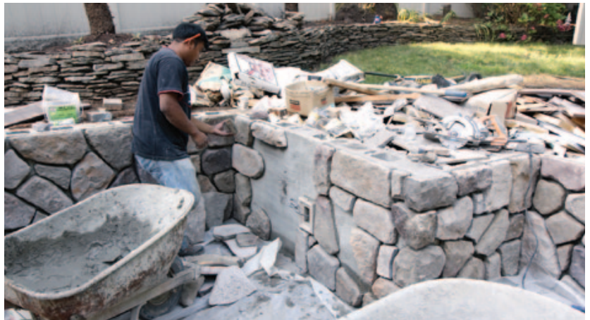
Figure 10. After the decking was complete, cultured stone was applied to the retaining wall.
