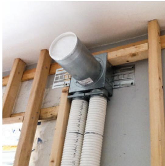
Figure 5. An air-sealed layer of XPS in the downstairs ceiling minimizes heat loss to the upstairs unit (above left). The exterior walls of the first-floor apartment were also furred out with 2x3s to provide room for additional cellulose, as well as space for the HRV ductwork (above). To tighten the wall assembly even more, the author used an airtight drywall approach, installing receptacle boxes inside airtight Lessco boxes (left).
