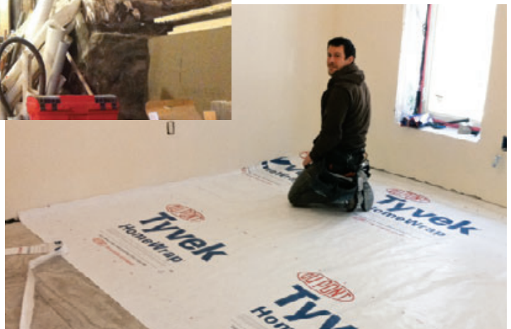
Figure 4. Working in the cellar, the crew applied foil-faced rigid foam to the bottoms of the first-floor joists, then sealed around the perimeter with spray foam; the joist cavities were later dense-packed (left). To further reduce air movement between the basement and living space, the author laid housewrap across the sub-floor above, taping the seams and sealing it to the drywall perimeter before laying the finish flooring (below).
