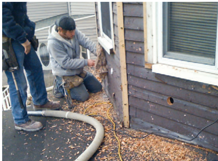
Figure 1. Because the original balloon-framed walls had never been insulated, dense-pack cellulose was easily blown into the empty stud cavities from the exterior.
