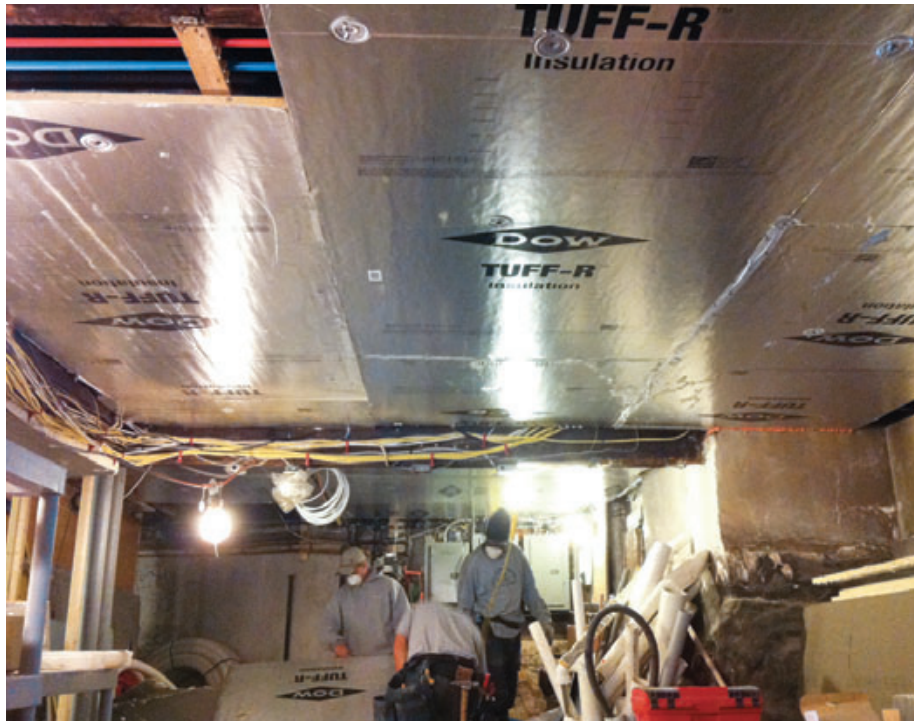
Figure 4. Working in the cellar, the crew applied foil-faced rigid foam to the bottoms of the first-floor joists, then sealed around the perimeter with spray foam; the joist cavities were later dense-packed (left). To further reduce air movement between the basement and living space, the author laid housewrap across the sub-floor above, taping the seams and sealing it to the drywall perimeter before laying the finish flooring (below).
