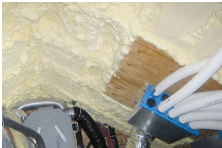
Figure 3. The roof framing in the attic mechanical room is encapsulated in a thick layer of closed-cell spray foam, bringing all the hvac equipment and ductwork within the building's thermal envelope. Plywood panels, fastened to blocking before the foam was applied, provided solid mounting surfaces where needed. To meet the fire code, the exposed foam was coated with intumescent paint.
