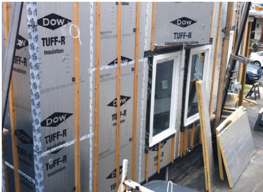
Figure 2. Energy-efficient casement windows were cantilevered beyond the original rough openings, secured with metal ties, then surrounded with snug-fitting rigid foam, which also serves as the wall's drainage plane.
