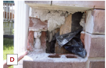
Figure 6. Destructive inspections from inside (A, B) and out (C, D) often reveal the cause of moisture, stains, and mold on interior finishes: The cavity is clogged with mortar, which holds water that eventually soaks the sheathing, framing, insulation, and drywall.
