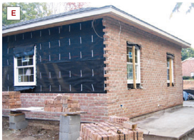
Figure 8. A durable job starts on a soldered copper base flashing (A), with the first course properly tied (B) and set on a weep cut from a Carlisle rubber traffic pad turned upside down, as seen in this photo from another job (C). The cavity is kept clean (D), and ties are spaced every 2 feet vertically and securely attached to the studs with galvanized ring-shank nails (E).
