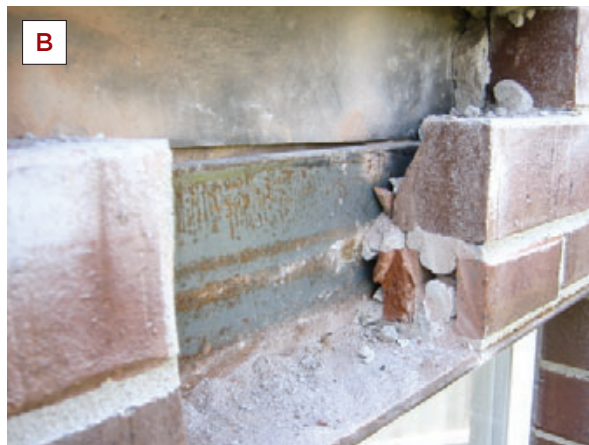
Figure 4. The rubber flashing tape intended to direct water onto the steel lintel (A) has pulled away from the housewrap and is instead directing water into the framing. Here (B), a metal flashing above the window just misses the lintel. Note the amount of mortar clogging the cavities in both cases. At left (C), a failed job required all the brick to be removed, revealing improperly flashed lintels at the windows, as well as ties that were never used.
