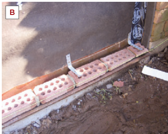
Figure 8. A durable job starts on a soldered copper base flashing (A), with the first course properly tied (B) and set on a weep cut from a Carlisle rubber traffic pad turned upside down, as seen in this photo from another job (C). The cavity is kept clean (D), and ties are spaced every 2 feet vertically and securely attached to the studs with galvanized ring-shank nails (E).
