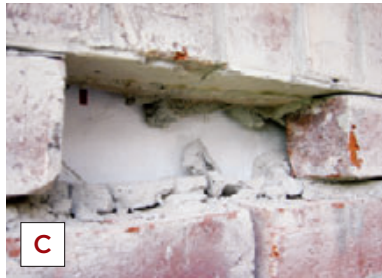
Figure 6. Destructive inspections from inside (A, B) and out (C, D) often reveal the cause of moisture, stains, and mold on interior finishes: The cavity is clogged with mortar, which holds water that eventually soaks the sheathing, framing, insulation, and drywall.
