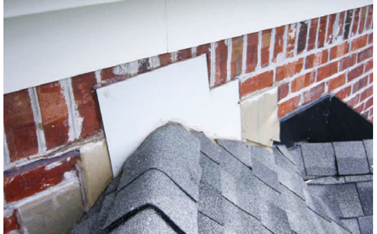
Figure 2. Stepped counterflashings installed in mortar joints (above) are no better than saw-cut flashings at diverting water from the cavity — unless they happen to run through to the sheathing and tuck under the building paper, which is rare. The work often gets sloppier where the installer thinks no one will see it, as in this bungled mishmash of surface-applied metal (right).
