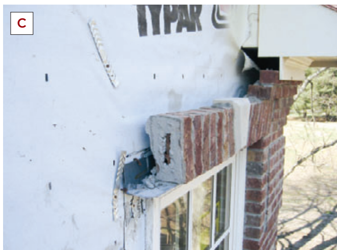
Figure 4. The rubber flashing tape intended to direct water onto the steel lintel (A) has pulled away from the housewrap and is instead directing water into the framing. Here (B), a metal flashing above the window just misses the lintel. Note the amount of mortar clogging the cavities in both cases. At left (C), a failed job required all the brick to be removed, revealing improperly flashed lintels at the windows, as well as ties that were never used.
