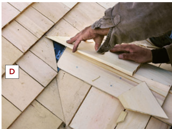
Figure 4. With the nail held back from the valley, the second starter pair is installed over flashing (A). The work continues in the same fashion up the valley, with a piece of metal under every pair of shingles (B). Where the valleys hit the main roof (C), metal flashing sealed with peel-and-stick rubber is applied, followed by a woven ridge cap (D, E).
