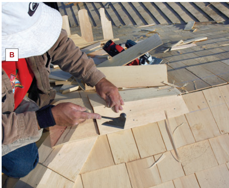
Figure 10. With the two hips capped, work proceeds along the ridge, where a double lap over the hip cap (A) is followed by alternating woven pairs (B). The results are classy (C, D).
