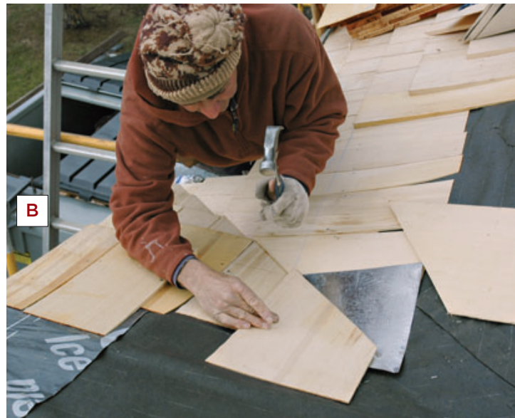
Figure 4. With the nail held back from the valley, the second starter pair is installed over flashing (A). The work continues in the same fashion up the valley, with a piece of metal under every pair of shingles (B). Where the valleys hit the main roof (C), metal flashing sealed with peel-and-stick rubber is applied, followed by a woven ridge cap (D, E).
