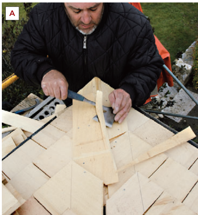
Figure 8. Hip caps are installed from alternating sides so that the joints don't align. The hatchet (A) and sometimes a block plane (B) are used to create smooth surfaces and trim the joints. A single exposed nail pins the sides together (C).
