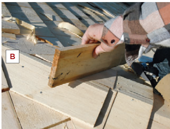
Figure 7. It's critical that woven hip caps lie tight to the shingles beneath, so spacers are used as needed (A) and the fit is constantly checked (B).
