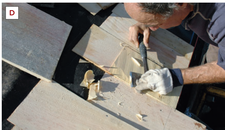
Figure 2. The author uses the gauge button on the shingling hatchet to lay out courses. The hatchet comes with button-holes every \frac{1}{2} inch; he heats the blade and uses a drill press to make additional holes at \frac{1}{4} -inch increments (A), which is enough to handle any spacing variations. The hatchet is much faster than wood strips for lining up courses (B), and is also the perfect tool for shaving shingles to even out inconsistencies in the roof plane (C, D).
