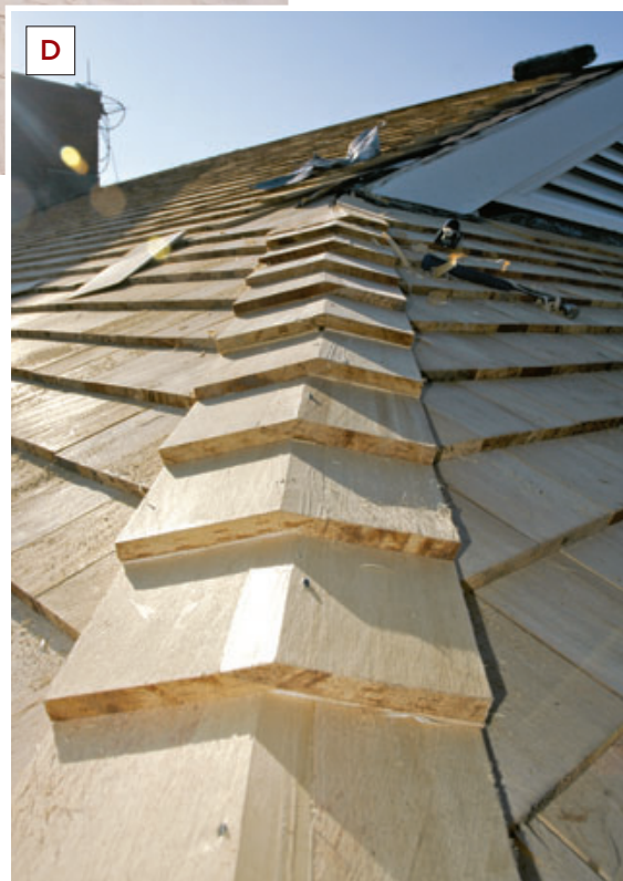
Figure 10. With the two hips capped, work proceeds along the ridge, where a double lap over the hip cap (A) is followed by alternating woven pairs (B). The results are classy (C, D).
