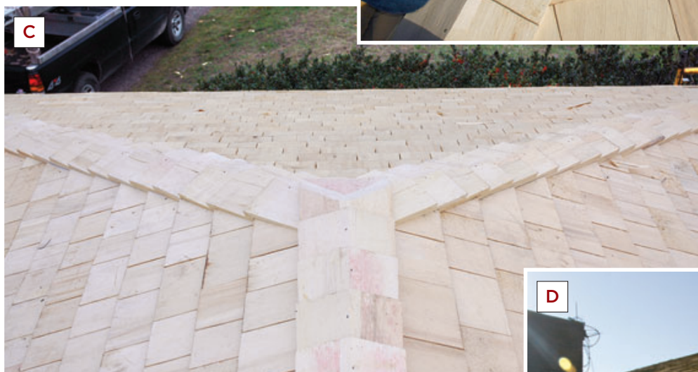
Figure 10. With the two hips capped, work proceeds along the ridge, where a double lap over the hip cap (A) is followed by alternating woven pairs (B). The results are classy (C, D).
