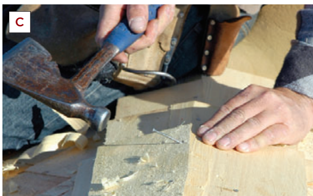
Figure 8. Hip caps are installed from alternating sides so that the joints don't align. The hatchet (A) and sometimes a block plane (B) are used to create smooth surfaces and trim the joints. A single exposed nail pins the sides together (C).
