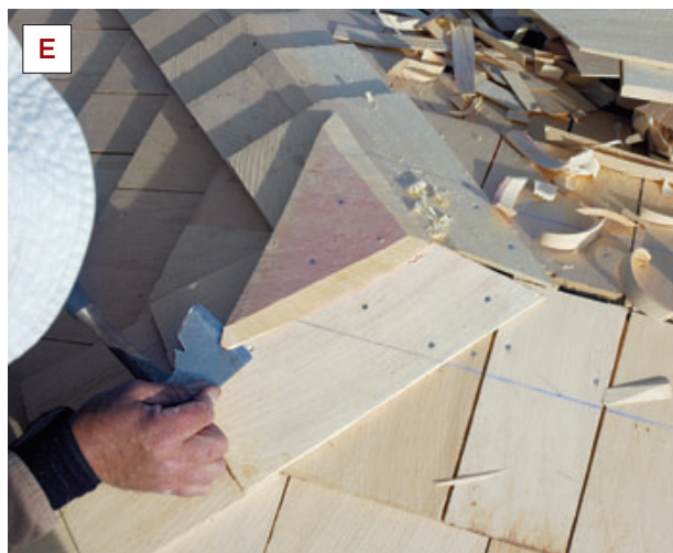
Figure 9. At the top, the hip runs on both sides are completed (A, B), then trimmed to the ridge line. A wide shingle (C), marked in place and cut to match the angle of the intersection (D), caps both sides (E).
