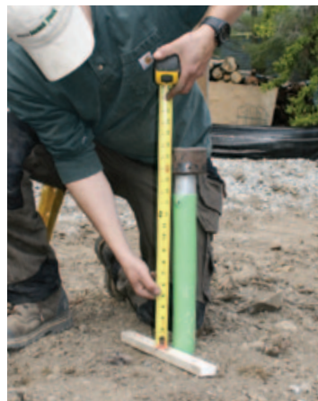
Figure 3. Shaft extensions are welded on and the pier driven as deep as needed to reach soil with adequate bearing capacity (A). The pier can be steered around a below-grade rock by moving the driver's boom; once the obstruction is passed, the boom pulls the shaft plumb again (B). Even though this pier penetrates about 13 feet into the ground, there's no pile of excavated soil as there would be with a conventional footing (C).
