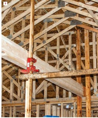
for far more weight than we'll ever lift. To locate choke points for the straps, we typically split a beam into thirds. The strap angle off the beam should be 60 degrees or greater. (Note: Some states may have specific rules about who can rig.)
