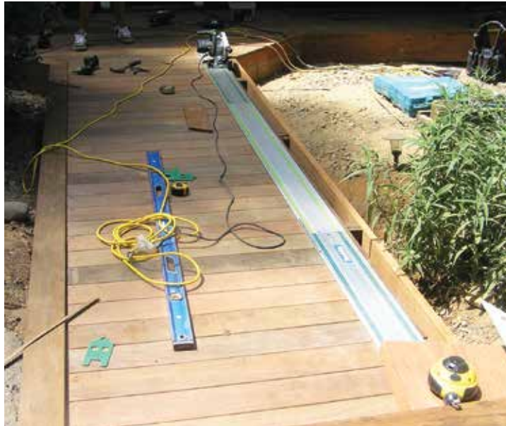
Figure 3. Makita and Festool tracks can be connected to make a very long rail. For even longer cuts, the author snaps a chalk line and aligns the track edge with the line. Clamps can be used to lock tracks in place but aren't usually needed thanks to soft rubber friction strips on the bottom of the tracks, which grip the cutting surface.
