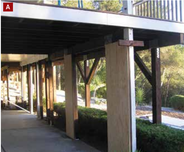
Figure 5. This unusual project required retrofitted posts tied to the existing posts with plywood sheathing (A). To create the mini shear walls, the author had to accurately rip the sheathing to size, a job that the track saw excels at (B). Once the track is in the proper position, the saw can be operated with either hand, with no loss in accuracy (C).
