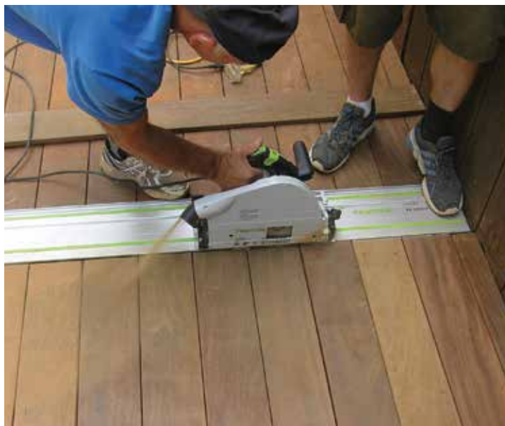
Figure 4. When decking meets decking at a slight angle, the author installs a saddle (right), which requires perfectly straight and parallel end cuts in the opposing decking. A little foot pressure is all that's needed to keep the track from slipping during the cut (left).
