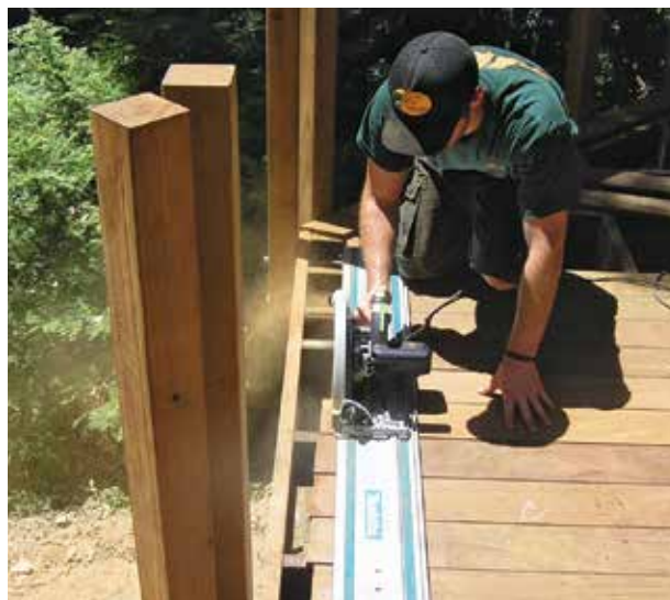
Figure 2. The Festool TS 75 EQ has a 2 \frac{3}{4} -inch cutting capacity; here it is being used to trim decking so that the deck can be picture-framed.
