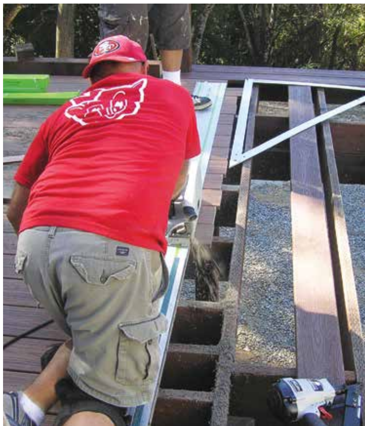
Figure 7. Trimming deck boards generates a large amount of sawdust. The dust-collection port isn't connected to a vacuum here, but if it were, the jobsite would remain virtually dust-free.
