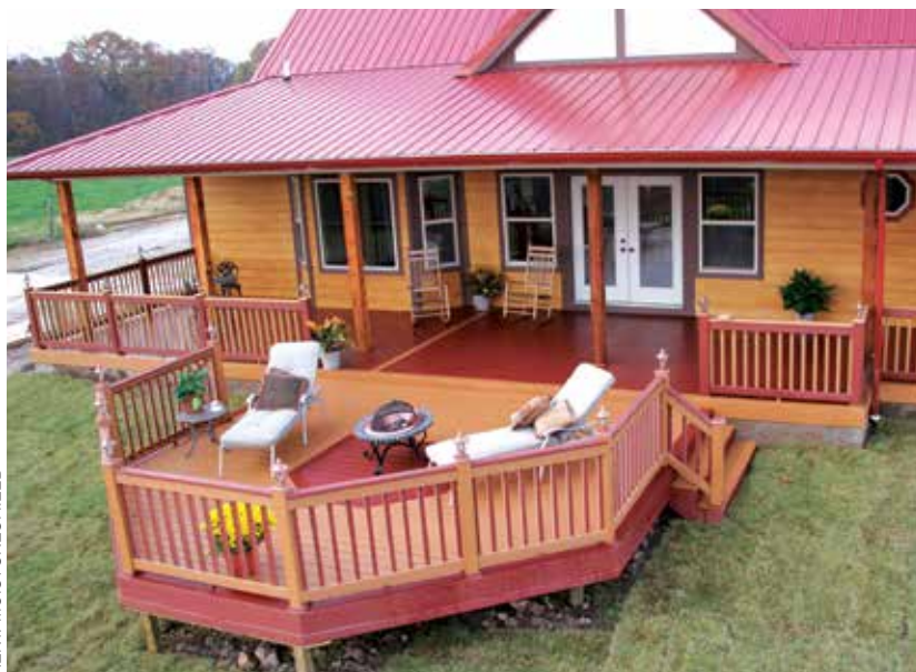
Figure 3. Many decking manufacturers offer railing systems that complement or match the colors of their decking. Usually rail parts are packaged separately, making it easy to match the balusters and rail cap with one color of decking, and the posts and rails with another, as shown with these MoistureShield composite products.
