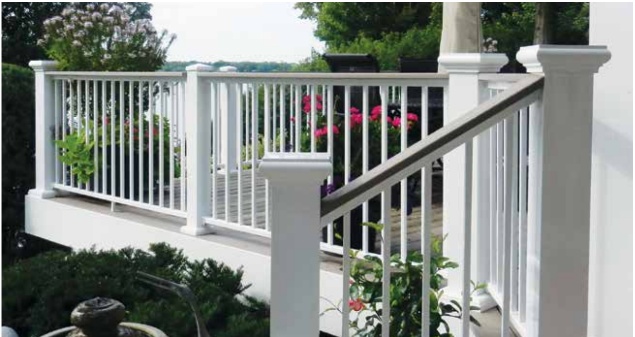
Figure 10. Fixed stair rail brackets are designed for standard stair runs of about 34 degrees, and usually offer a few degrees of variance. They're less expensive than adjustable brackets and faster to install, and have a lower profile.
