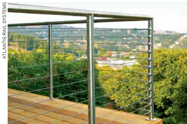
Figure 11. Horizontal cable rails are popular not only for their sleek, contemporary look but because the thin cables are almost invisible. Many cable-rail companies sell pre-engineered railing systems complete with surface-mounted posts and cable runs.
