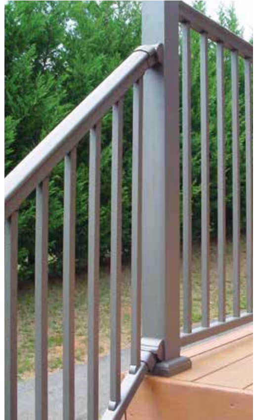
Figure 10. Fixed stair rail brackets are designed for standard stair runs of about 34 degrees, and usually offer a few degrees of variance. They're less expensive than adjustable brackets and faster to install, and have a lower profile.
