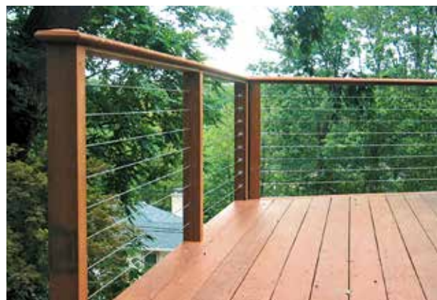
Figure 12. Cable balusters can be integrated into a wood rail system, though most manufacturers have special post installation requirements, such as separate posts at each corner. In-house design assistance is usually available from cable rail manufacturers to help engineer the railing.
