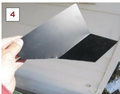
Many builders use plastic or metal kick-out flashings at the base of long roof sections to direct large volumes of water running down the roof away from the siding below. I find these flashings ugly and easily broken, however, so I try to avoid them. Instead — particularly for short roofs that are more protected from the weather — I use a low-profile flashing detail that directs water to the front face of the siding, where it does no harm as it flows down the building.
