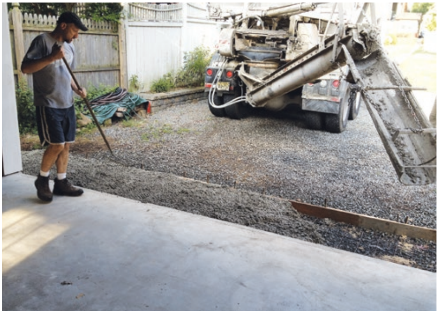
Figure 9. The apron slab was reinforced with wire mesh and sloped down toward the driveway 1 inch over its 4-foot width.
