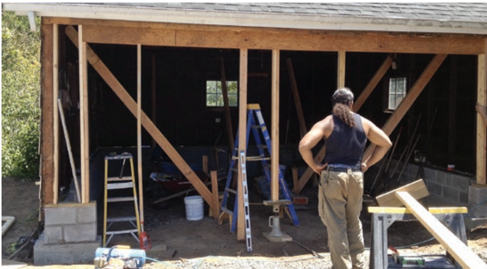
Figure 7. The wider overhead door required the installation of a double 11 7 / 8 -inch-deep Microllam header under the existing 4x4 top plate. A screw jack was used to level the opening and to support the beam until jack and king studs could be installed.
