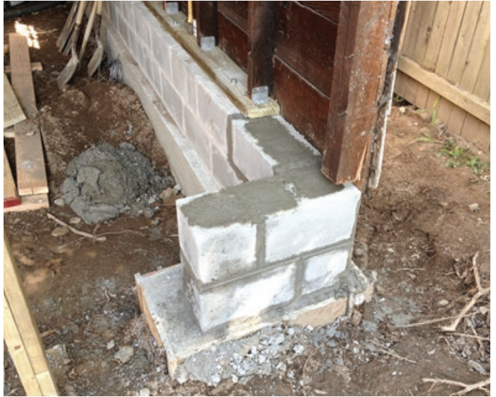
Figure 6. Like the rear footing, the front wall footing returns were pinned to the new gable-end footings with two #5 rebars (above), and the blocks were toothed together at the corner (right).
