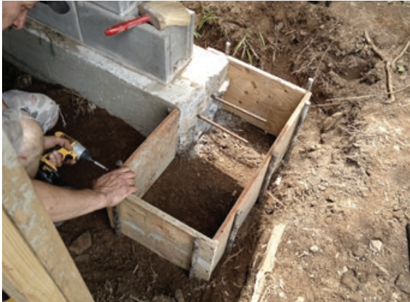
Figure 6. Like the rear footing, the front wall footing returns were pinned to the new gable-end footings with two #5 rebars (above), and the blocks were toothed together at the corner (right).
