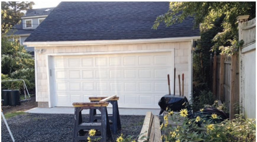
Figure 10. The bulk of the exterior finishes are on the front wall; new siding flanks a car-and-a-half-wide garage door (above). The exposed block stem wall was parged with mortar, and the driveway was regraded with new gravel. Gutters were added, and a berm was created to help direct runoff away from the entry apron (left).
