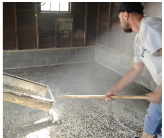
Figure 8. After laying down a layer of 4-inch gravel, reinforced 6-mil poly sheeting, and welded-wire mesh, the crew ran asphalt-impregnated fiberboard around the inside face of the footing (left), then poured the new 4-inch slab flush with the top of the footing (right). The fiberboard serves to isolate the slab from the footing should any frost issues arise.
