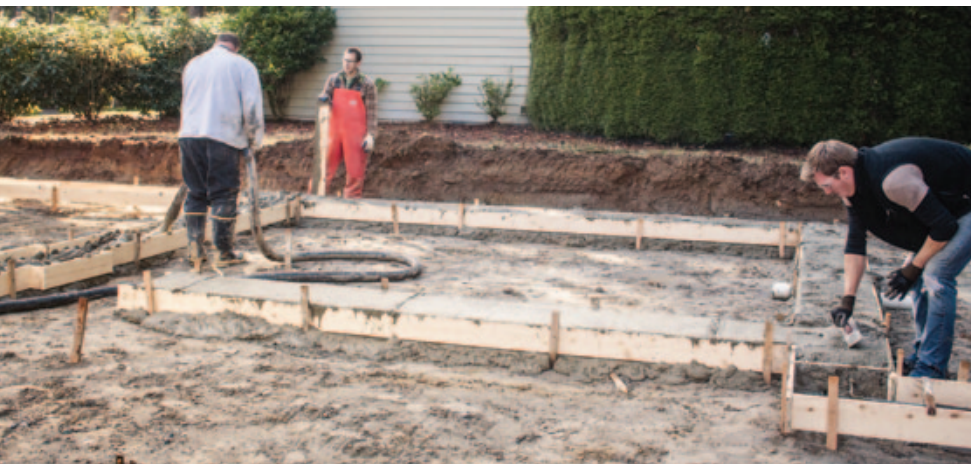
Figure 11. As the line pump operator fills the footing form, a crew member follows behind and screeds the concrete level. A second worker then trowels the footing smooth.
