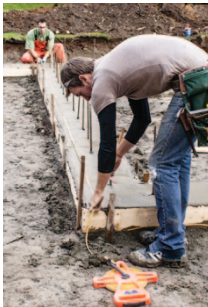
Figure 12. Workers lay out the stem walls on the footings, snapping lines while the concrete is still soft.
