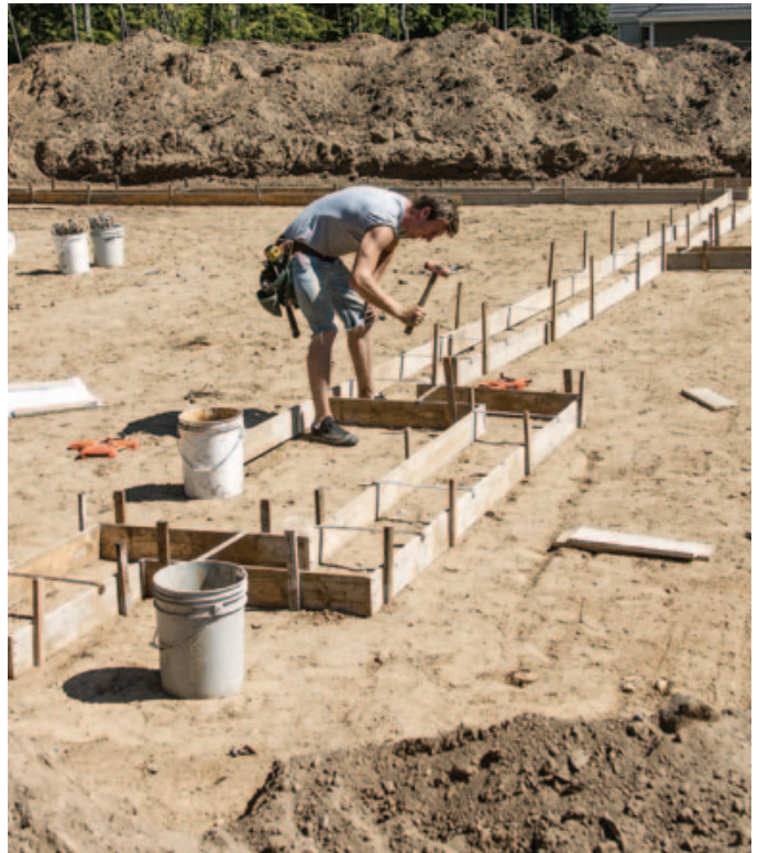
Figure 3. Either metal or wooden stakes can be used to hold the forms in place. In hard ground, a metal stake can be used to “predrill” holes for cheaper wooden stakes.
