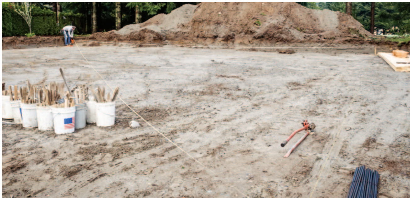
Figure 1. When laying out the footings, the author determines diagonal measurements using the rise/run function on his construction calculator, then refers to those measurements to verify that corners are square. The stretched string on the right-hand side of the photo indicates the outside edge of the first set of footings.
