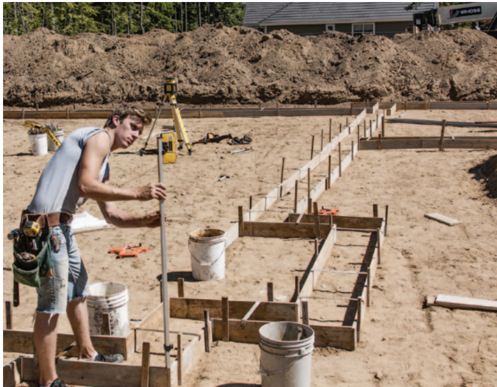
Figure 4. A single crew member can level the staked forms using a rotary laser. The receiver included with the Stabila LAR250 kit used by the author indicates distance from grade in \frac{1}{16} -inch increments.
