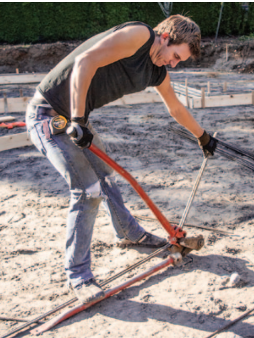
Figure 7. Most contractors cut and bend rebar on site, as shown. An option in some areas is to have a local metal shop pre-cut and pre-bend the rebar.
