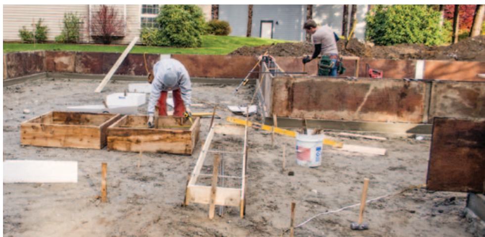
Figure 10. Here, the author's crew has formed footings for an interior shear wall and for several large piers that will support point loads from the roof.
