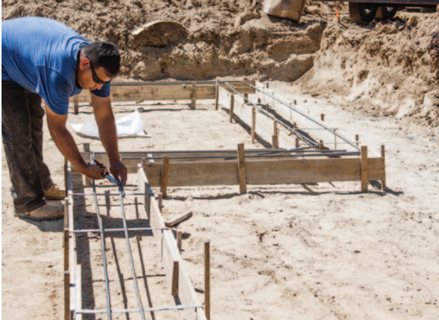
Figure 5. Tying the rebar together on top of the spreader cleats makes it easier to get the overlaps and spacing right. Afterward, the spreaders can be temporarily removed and the rebar dropped in place.
