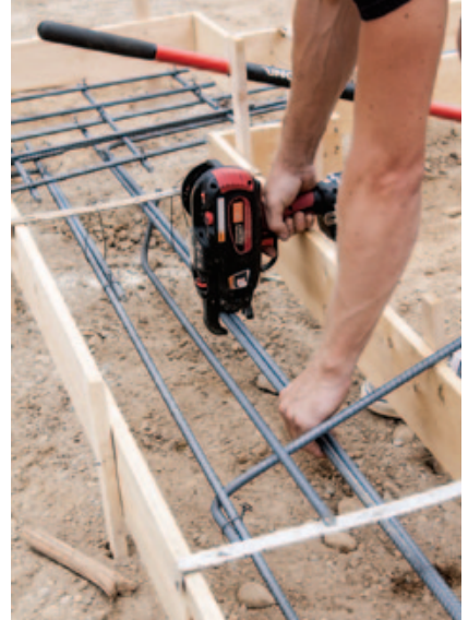
Figure 6. Companies that do production foundation work may want to consider the Max cordless rebar tier ( maxusacorp.com ), which automatically makes a tie in less than a second.
