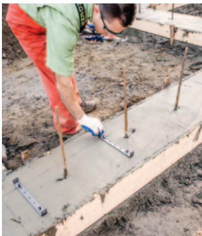
Figure 13. Form clips are set every 16 to 24 inches along the snapped layout lines. The author holds them in place with 1½-inch Teco nails pushed into the wet concrete; even if rain washes the lines away, the clips will still be in the right position for the stem-wall forms.
