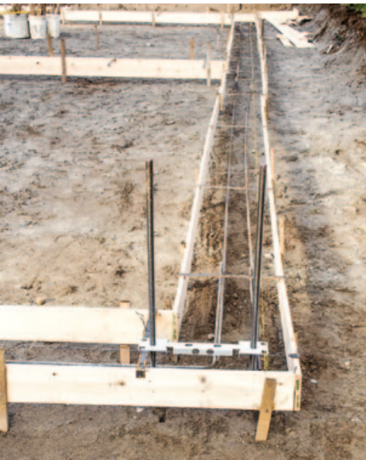
Figure 8. To place the rebar at the proper depth in the footing, the author suspends it from the spreader cleats. Here, he's also used a template to accurately locate the 1-inch-diameter all-thread rod needed for an iLevel shear-wall brace.
