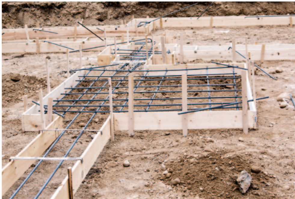
Figure 9. Areas in the footings that must support point loads are reinforced with rebar following the engineer's specifications.
