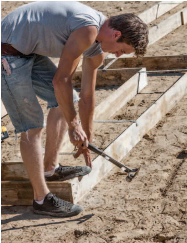
Figure 2. Footing forms are fastened together at the corners with duplex nails; 16-inch metal spreaders keep the sides properly spaced.
