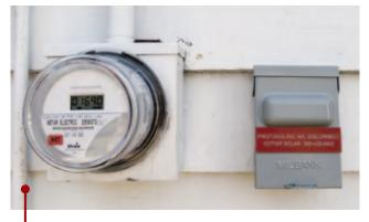
10. A second meter on the outside wall registers the homeowner's net power use, spinning forward or backward depending on whether the home is drawing power from the grid or supplying it. If more power is produced than used, there's no electric bill that month. A utility-required emergency shutoff switch allows utility workers to confirm that the panels are offline when needed.
