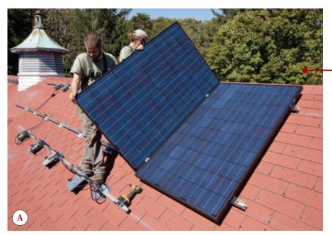
8. Starting at one end of the mounting rails, workers move modules into position and connect their positive and negative leads to the microinverter input fittings (A). Cables are zip-tied to the rails or module frames as needed to prevent them from rubbing against the shingles or trapping debris (B). Another set of mounting clips is positioned against the outside edge of the module frame, and the sequence is repeated for the next module (C).
