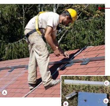
2. After snapping lines marking the position of the rafters, the installer lays out the first extruded-aluminum mounting rails, which will be fastened to each rafter with a 5/16-inch hot-dipped lag screw (A). The rails are held off the roof at each connection by a short spacer or "mounting foot" cut from extra railing material (B, C). A manufactured aluminum flashing tab (D) is slipped under the shingle above; its rubber grommet forms a weatherproof seal around the lag.
