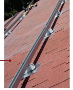
**3.** Where required, rail sections are joined between mounting feet with splice fittings that allow for necessary thermal expansion and contraction. The fittings add enough flexibility to allow the rails to conform to minor irregularities in the roof plane.
