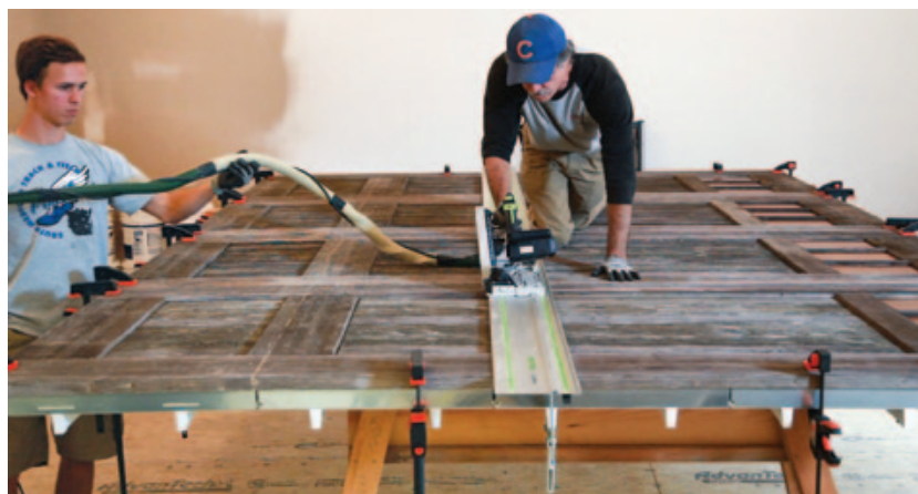
Figure 6. The author cut through the carriage doors using a track-mounted saw for accuracy (above). The blade was set with a slight 2-degree bevel for drainage (left).
