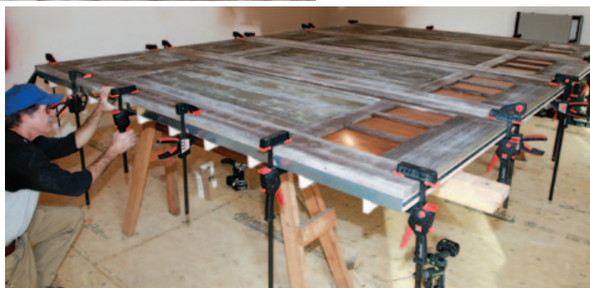
Figure 5. Once the carriage doors were assembled, the author spread construction adhesive on the steel door panels (left), then clamped the carriage doors in place (below). Dozens of 3-inch self-tapping coated screws driven through the backs of the roll-up panels into the stiles and rails of the carriage doors join the wood and steel door sections together.
