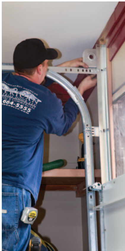
Figure 7. The door company used special track-mounting hardware to accommodate the 3\frac{1}{4} -inch-thick door (above). Each of the five roll-up panels weighs 120 pounds (above right), but the assembled door (right) is easily operated by one person, thanks to the commercial-style coil spring counter-weight mechanism.
