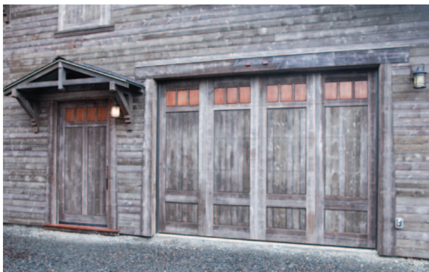
Figure 7. The door company used special track-mounting hardware to accommodate the 3\frac{1}{4} -inch-thick door (above). Each of the five roll-up panels weighs 120 pounds (above right), but the assembled door (right) is easily operated by one person, thanks to the commercial-style coil spring counter-weight mechanism.
