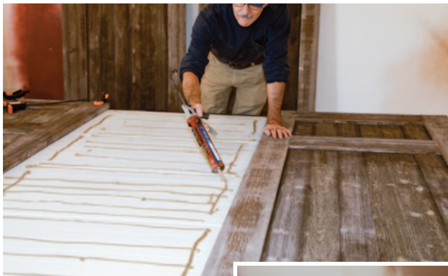
Figure 5. Once the carriage doors were assembled, the author spread construction adhesive on the steel door panels (left), then clamped the carriage doors in place (below). Dozens of 3-inch self-tapping coated screws driven through the backs of the roll-up panels into the stiles and rails of the carriage doors join the wood and steel door sections together.
