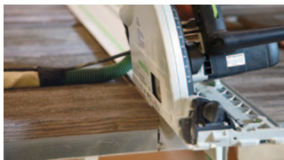
Figure 6. The author cut through the carriage doors using a track-mounted saw for accuracy (above). The blade was set with a slight 2-degree bevel for drainage (left).
