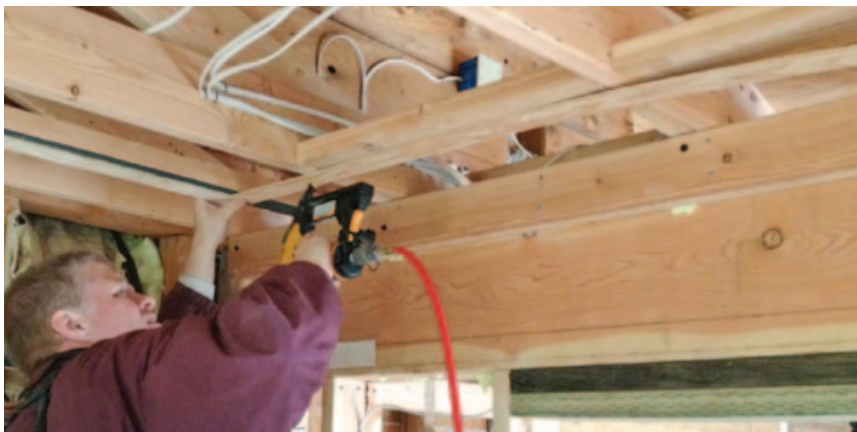
Figure 3. To bring the \frac{5}{8} -inch ceiling drywall, \frac{1}{2} -inch wall drywall, and \frac{1}{4} -inch flexible drywall that would be used to form the cove into the same plane, \frac{1}{4} -inch plywood furring strips needed to be attached to the blocking.
