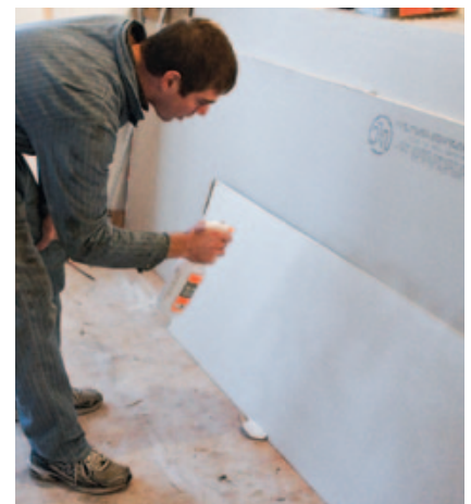
Figure 6. Workers sprayed both sides of each panel with a mister. Allowing the wet panels to sit for a few minutes before installation increased their flexibility even more, making it easier to form the flexible drywall to the 12-inch radius of the cove.
