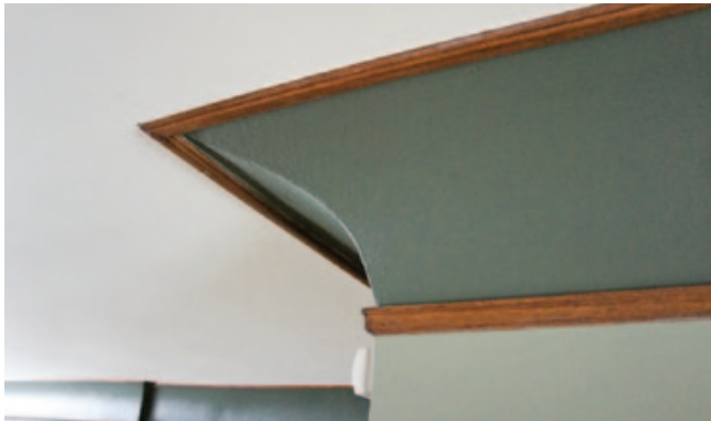
Figure 1. The ceilings in the original house had an interesting cove detail (above) that the homeowners wanted to duplicate in their new addition, but with typical drywall instead of traditional plaster-and-lath construction (right).
