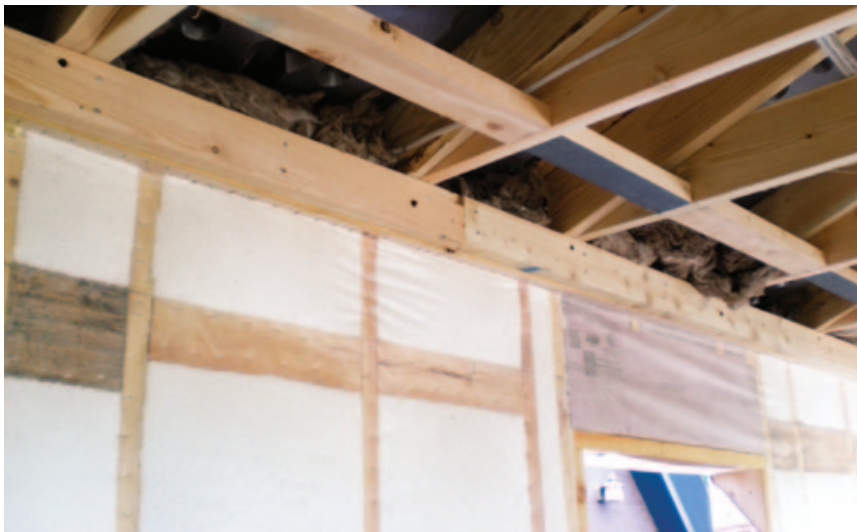
Figure 2. To provide a solid attachment point for the prefabricated arches, the author installed rows of blocking between the wall and ceiling framing. The blocking is centered 12 inches from the wall/ceiling intersection, and also provides good backing for drywall.
