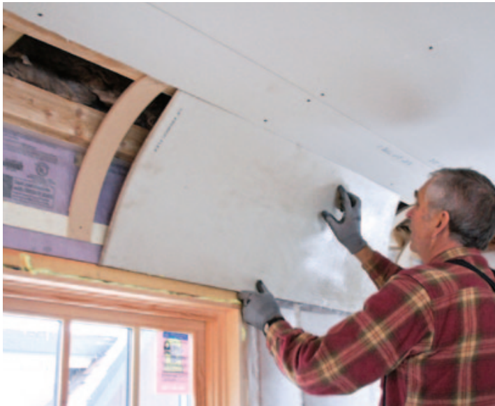
Figure 7. When forming the panels, crewmembers worked slowly and avoided pushing hard on the center of the panel, which would break the paper face and buckle the drywall (above). Once the panels conformed to the cove, they were screwed in place with regular drywall fasteners on 5-inch centers (right).
