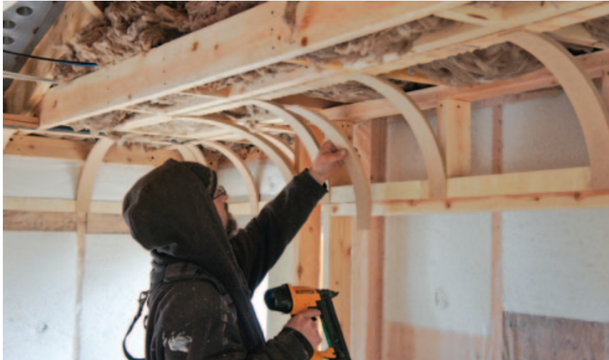
Figure 4. The arches were fastened to the furring strips 16 inches on-center. A narrow crown stapler and dabs of construction adhesive were used to make the attachment.
