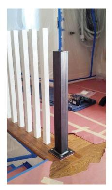
the newel off, drilled holes for lags, and anchored it down. I lathered up the stanchion with PL Premium about three-quarters of the way down from the top, and added a healthy dose right at the weld joint area. I carefully slipped the newel over, and propped a stick against the ceil-
