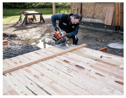
With the Big Foot Head Cutter (a saw table for a chain saw), the author makes 33 tail cuts in a single pass through a bundle of I-joist rafters. The whole process — including racking, layout, and cutting — took about 30 minutes.
