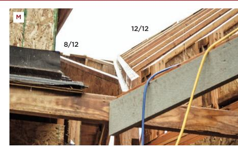
the LVL on that side square, while on the 12/12 side we ripped a bevel to match the steeper slope. Working from a section drawing (N), we were able to measure how much we had to build up the plate to support the 12/12 rafters (O). Doing it this way meant the bottom of the valley would have a crisp edge that matched both slopes, making a perfect surface on the inside where the two drywall planes join.
