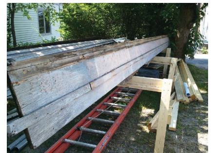
Figure 1. Before the renovation, the building was essentially sound, but the years had not been kind to it. Asbestos shingles covered the walls (left), and much of the trim had deteriorated beyond saving. As the exterior layers were peeled back, any of the original cypress trim that still had life was set aside to be reinstalled later (above).
