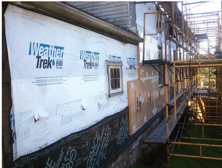
Figure 2. Before the nailing strips went on, cellulose insulation was blown into the walls; housewrap was attached to the original sheathing (above) to keep the cellulose from leaking out. Then the walls were wrapped with foil-faced foam and the seams taped. Vertical strapping was screwed through the foam and into the framing to attach the siding and trim (left). Extra stock was later added around window and door openings for nailers. Vent strips were installed at the top and bottom of each wall for drainage and to allow air to flow freely behind the clapboards (bottom).
