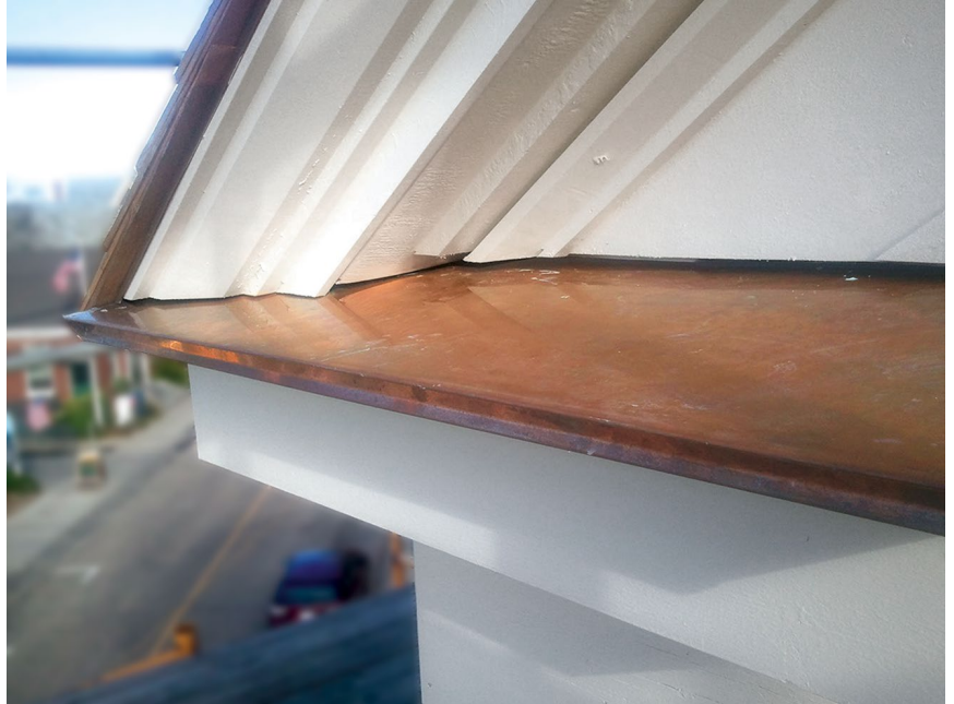
Figure 4. When the trim went back on the building, original detailing was followed as closely as possible based on archival photos and the trim that was removed (above). Metal connectors and beams were added where the old structure needed strengthening (left).
