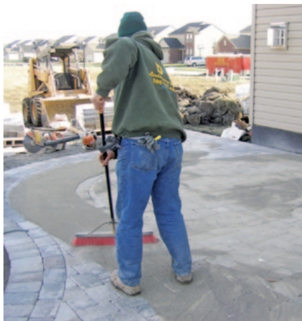
Figure 12. Mason sand swept across the finished surface fills the joints between pavers.
