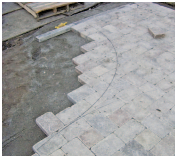
Figure 9. For many curves, the author lays the pavers beyond the line of the curve and cuts them in place.
