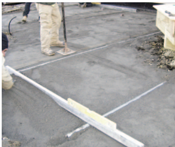
Figure 3. Lengths of one-inch-diameter conduit are set into the compacted base to serve as screed guides (top). After adding stone around the guides, the crew screeds and tamps the surface (bottom).
