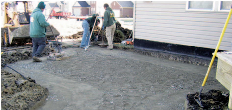
Figure 2. Crusher run stone laid in 3- or 4-inch lifts forms the base layer.
