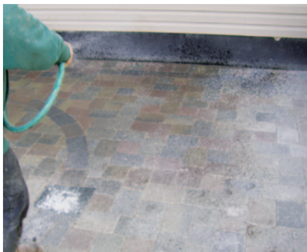
Figure 13. Though it should be installed in bone-dry conditions, wetting polymeric sand in place initiates a reaction that turns it into a flexible mortar. On some materials, however, it can leave a visible haze.
