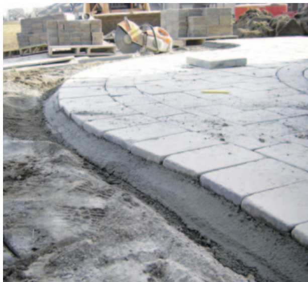
Figure 11. Mortar trowelled along the edge of the soldier course serves as an edge restraint. The author has found that this detail holds up well to freeze-thaw cycles.
