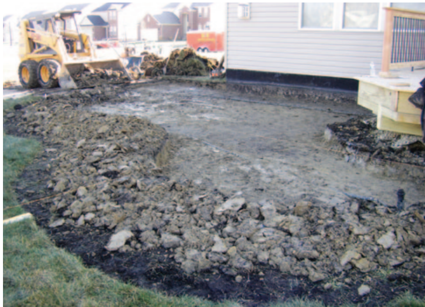
Figure 1. Every paver installation starts with excavating down to stable soil. Any unsuitable fill is removed and its replacement compacted to ASTM standards.
