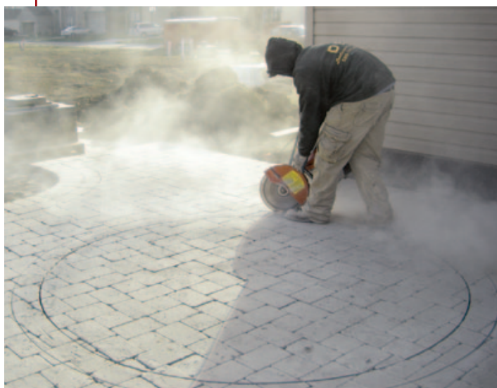
Figure 10. To create clean borders for inlays, all field pavers are set and compacted, then the pattern is cut out.
