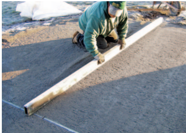
Figure 4. Smaller, \frac{3}{4} -inch-diameter conduit laid directly on the compacted base guides screeding of a concrete-sand bedding layer.
