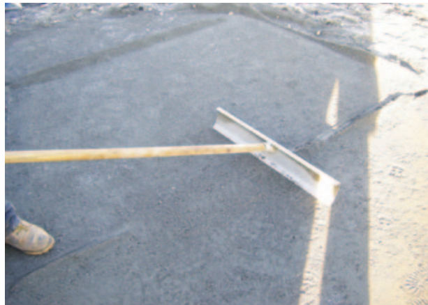
Figure 5. Before laying pavers, the crew removes the screed guides and fills the resulting troughs in the bedding layer with sand.
