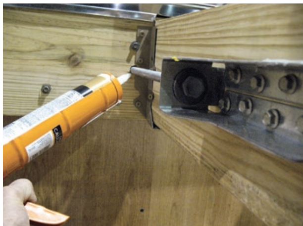
Figure 4. To keep out water and insects, the author caulks all holes drilled through the house. Note that he installs the brackets 6 to 8 inches away from ledgers, rims, and other framing members. The distance makes it easy to caulk holes in the rim joist, as well as access the brackets with a wrench or drill.
