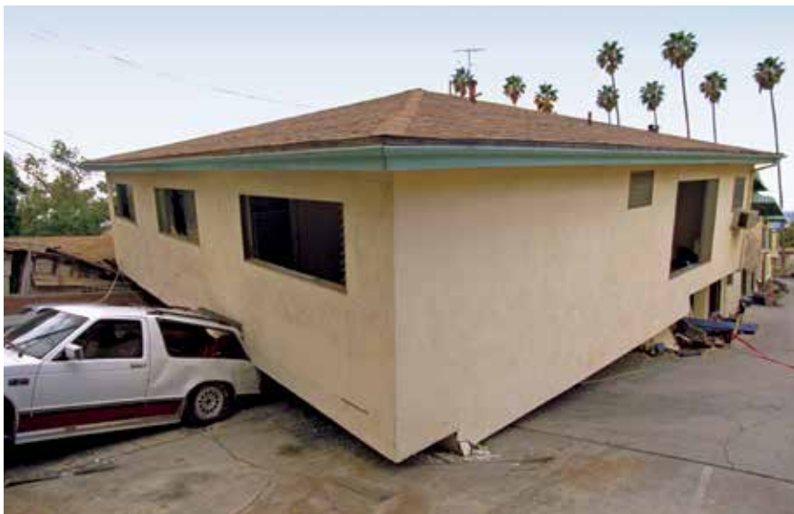
In an earthquake, shear walls help upper stories stay connected to the foundation, which moves rapidly back and forth. Without them, the movement gets too far out of sync, and the building "pancakes," as in this 1994 photo from Northridge, Calif.
