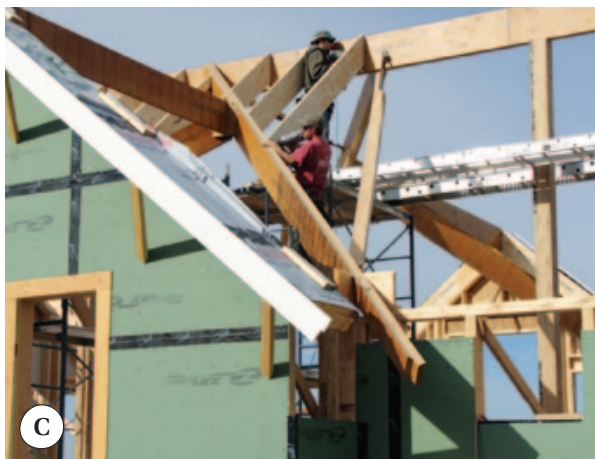
Figure 6. Since beveled valley rafters aren't a JobPack option, the author got these LVLs from his local lumberyard and cut them on site (A, B). The valley jack rafters were precut, but needed to be trimmed to size because of layout changes in the rest of the roof framing (C).
