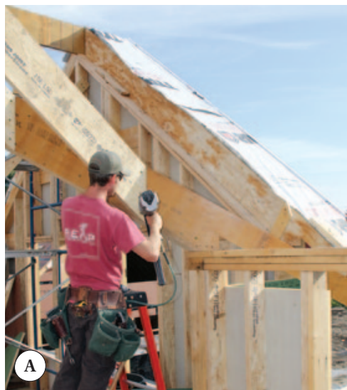
Figure 6. Since beveled valley rafters aren't a JobPack option, the author got these LVLs from his local lumberyard and cut them on site (A, B). The valley jack rafters were precut, but needed to be trimmed to size because of layout changes in the rest of the roof framing (C).
