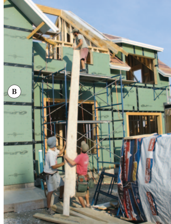
Figure 7. Some of the common rafters had to be cut on site from stock material (A). LSLs are a lot heavier than I-joists or sawn lumber; wrestling the 20-foot-long common rafters into position was a three-man job (B). Crew members tacked the dense material in place with a nail gun (C), then used impact drivers to drive structural screws through the rafters into the framing.
