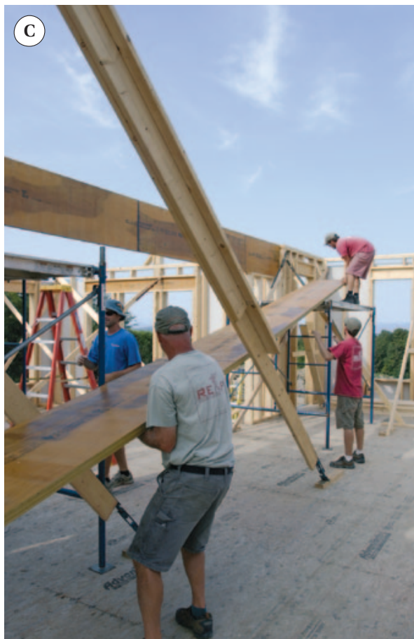
Figure 4. Once the first-floor walls were in place, the crew could install the second-floor support beams (A). While many of the beams were precut (B), a large 5 \frac{1}{4} -inch-wide by 24-inch-deep by 28-foot-long beam built up from three 1 \frac{3}{4} -inch by 24-inch LVLs was not, which allowed the crew to verify the length of the span, then cut and fit the beam one ply at a time (C).
