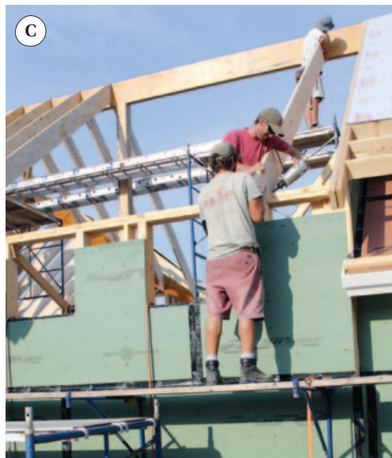
Figure 7. Some of the common rafters had to be cut on site from stock material (A). LSLs are a lot heavier than I-joists or sawn lumber; wrestling the 20-foot-long common rafters into position was a three-man job (B). Crew members tacked the dense material in place with a nail gun (C), then used impact drivers to drive structural screws through the rafters into the framing.
