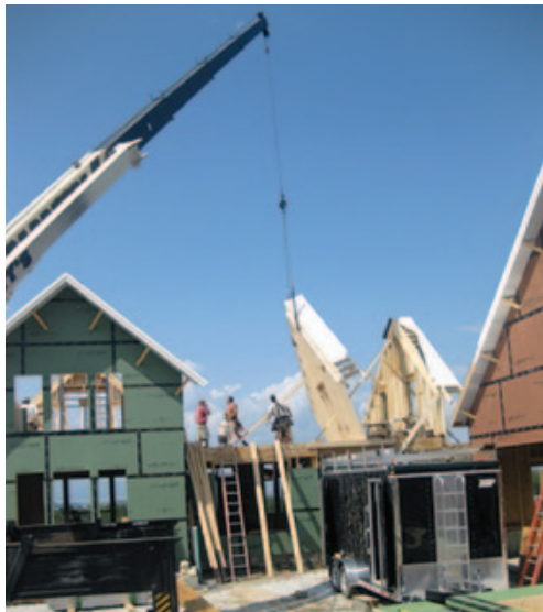
Figure 5. A crane was used to lift into place the panelized second-floor walls, including two rake walls with prefabricated eaves (right) and a major interior bearing wall (far right).
