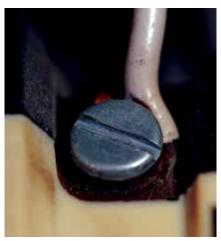
wire keeps it from carrying the fault current adequately, so the breaker won't trip as quickly as it is designed to, which can lead to a fire.
