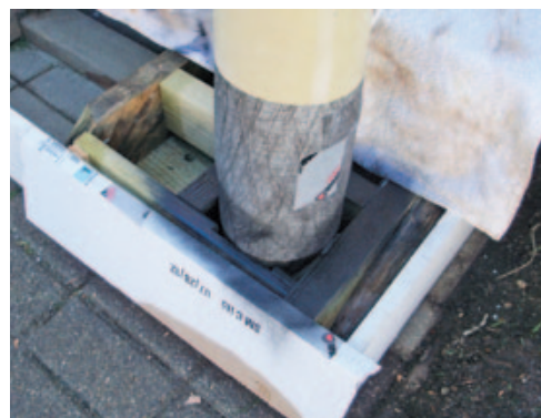
Figure 10. Black spray paint made the frame and lower part of the newel practically invisible once the tread boards were installed.
