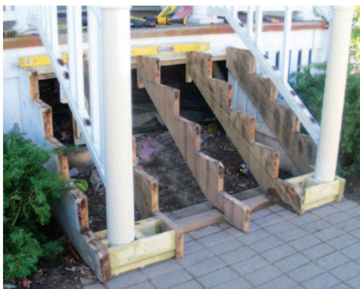
Figure 2. A pressure-treated frame was built to support the new posts and bottom tread.
