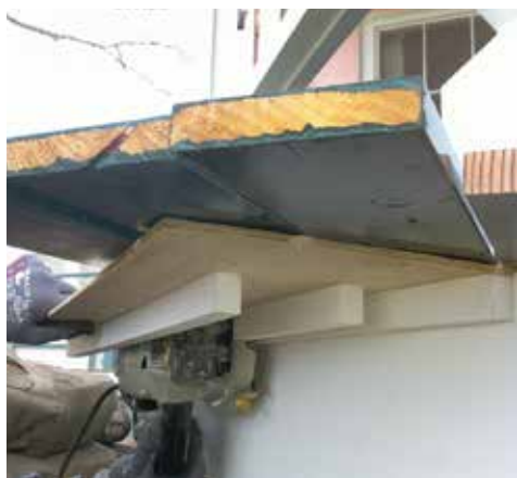
Figure 4. To cut the new decking to length after installation, the author made a plywood extension fitted with a curved fence for his Porter-Cable 4\frac{1}{2} -inch trim saw (left). One person manned the saw while another crew member removed the off-cuts (above).
