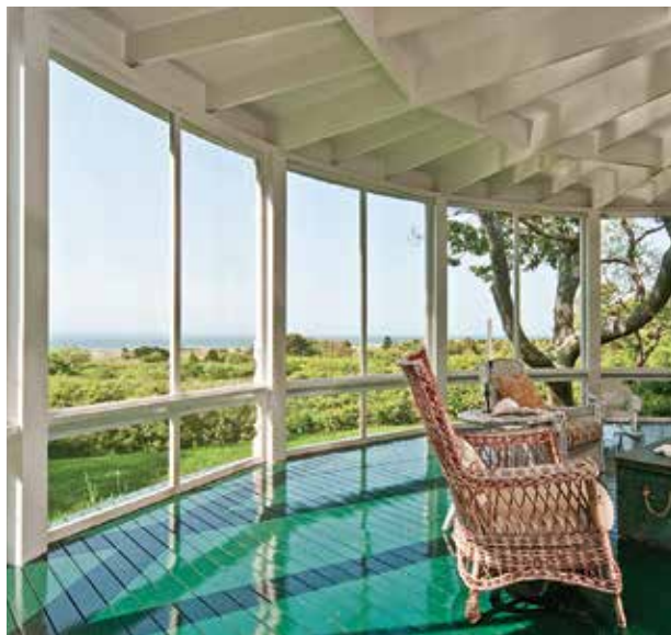
Figure 5. Documenting the existing ceiling height and panel dimensions before deconstruction made it much easier to reproduce the original appearance of the porch when it came time to put everything back together (top). The new vertical-grain fir decking for the refurbished porch was pre-finished with a durable marine topside paint (above).
