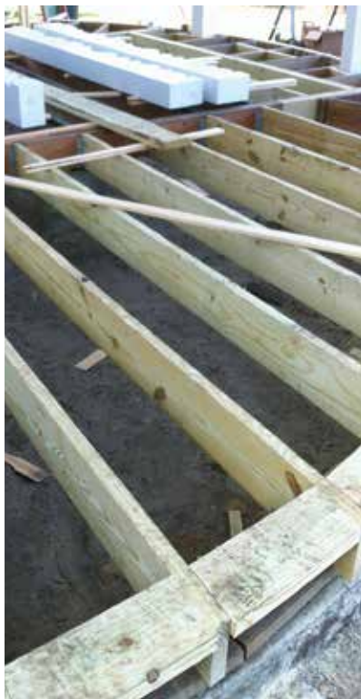
Figure 3. The author replaced the rotted joists with treated framing, then used a trammel arm (above) to scribe the deck's radius onto blocking installed on the flat around the perimeter of the deck (right).
