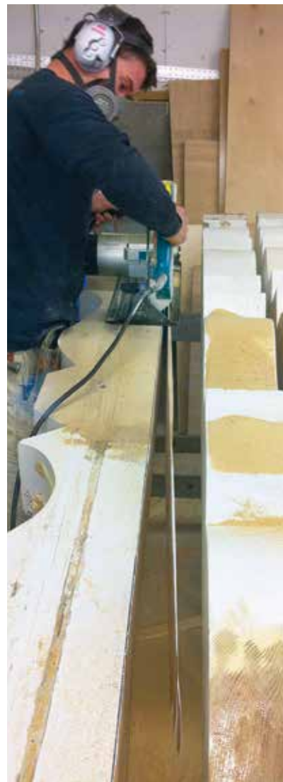
Figure 2. The new and old column sections were joined together with galvanized through-bolts and epoxy (left). Once the columns were reassembled, a worker straightened them with a large-capacity beam saw (right).
