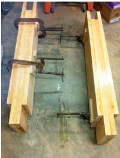
Figure 1. The 2x10 fir laminations of the partial replacement posts are offset to create a slot for joining to the original post sections (top left). After scribing the original column patterns (bottom left) and cutting them out on a band saw, the author created a matching tongue profile with a router (bottom right).
