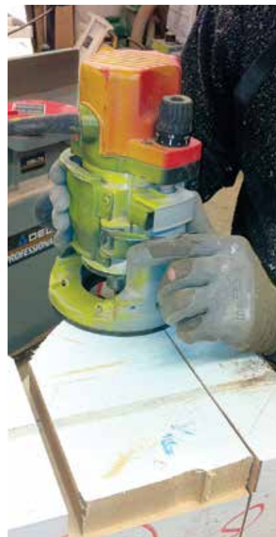
Figure 1. The 2x10 fir laminations of the partial replacement posts are offset to create a slot for joining to the original post sections (top left). After scribing the original column patterns (bottom left) and cutting them out on a band saw, the author created a matching tongue profile with a router (bottom right).
