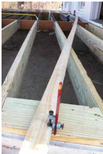
Figure 3. The author replaced the rotted joists with treated framing, then used a trammel arm (above) to scribe the deck's radius onto blocking installed on the flat around the perimeter of the deck (right).
