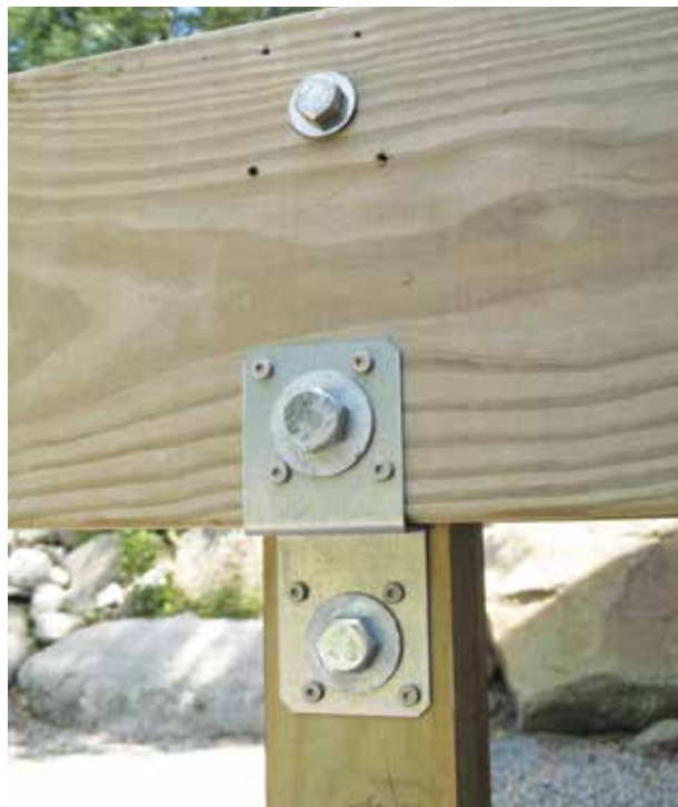
Figure 6. On 4x4 posts, metal hardware—including Simpson Strong-Tie's DJT14Z (shown) and USP's SDJT14-TZ—can be used to support side-applied beams.
