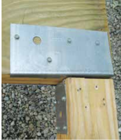
Simpson Strong-Tie EPC44 Medium-duty 12-gauge end-post/beam connector for 4-by posts
