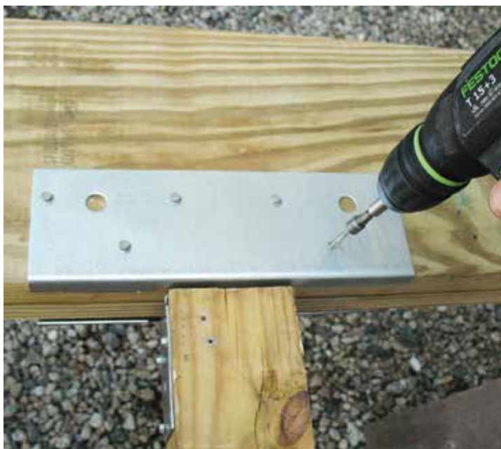
Figure 7. Using structural screws instead of nails will increase the uplift and lateral-load-bearing capacity of most metal connectors.
