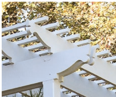
Figure 6. A general rule for the length of an overhang on an arbor is to double the nominal width of the lumber. For instance, a 2x8 joist should extend 16 inches beyond the beam it rests on. The author cuts decorative shapes on the trellis ends with a jigsaw and finishes them with a belt sander.
