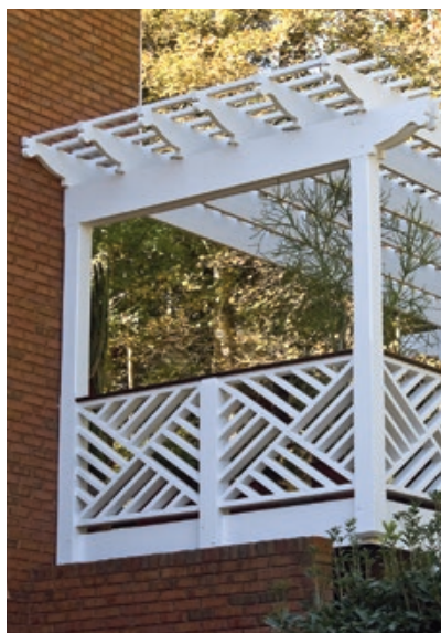
Figure 4. Even a single connection point to a house adds stability to an arbor.
