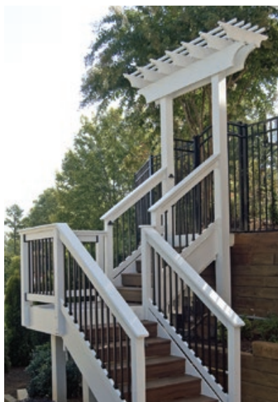
Figure 5. A freestanding arbor gains extra support from its attachments to railings and adjacent framing.
