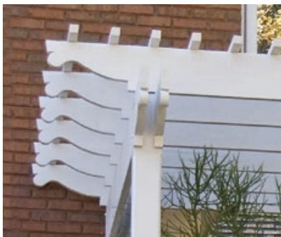
Figure 6. A general rule for the length of an overhang on an arbor is to double the nominal width of the lumber. For instance, a 2x8 joist should extend 16 inches beyond the beam it rests on. The author cuts decorative shapes on the trellis ends with a jigsaw and finishes them with a belt sander.
