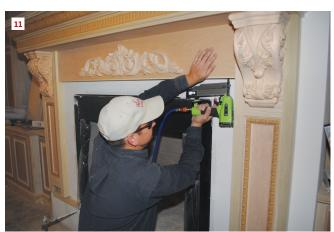
We added another strip of plywood on top of the first tier for attaching the second tier. I tacked the strip in place, and then checked the overhang of the plywood on all sides to make sure the reveals were even.
