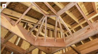
I do all the layout on this piece of sheathing, using its edges as the inside face of the 2x12 soffit, and drawing a diagonal across the corner to define the 67.5° corners where the hips will be nailed. A regular hip splits a 90° corner (making 45° angles); an octagonal hip then splits the 45° angle, making 22.5° angles between the hip and the commons on either side of it.
