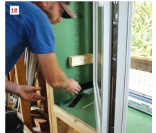
The bolted connection is quick and simple to make and has the advantage of holding the window in position front to back as well as from side to side (the positive thread connection means the windows couldn't rack—even without the shims). Also, the bolts don't get in the way of air-sealing and insulating: The crew will first inject foam sealant into the gap, then trim the foam on the inside and tape the window face to the inside buck before drywalling the opening.
