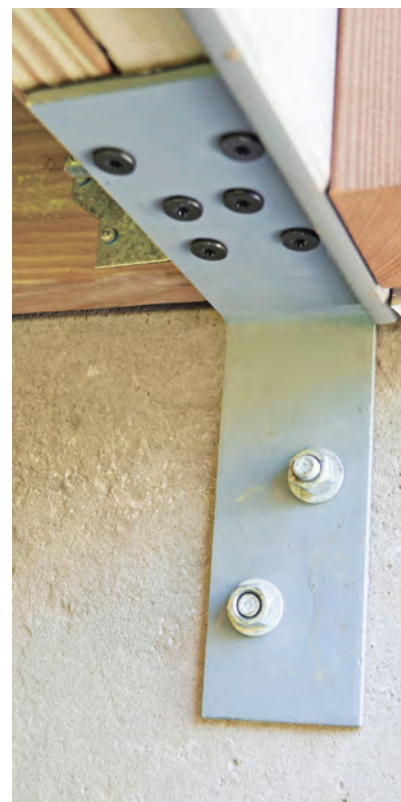
Figure 3. The author designed a second custom L-bracket for use without a 2-by brace. It's fabricated from ¼-inch-thick steel plate, with each leg measuring 3 inches by 9 inches. The brackets are hot-dipped galvanized for corrosion protection, and when installed, are isolated from treated framing with self-adhering flashing.
