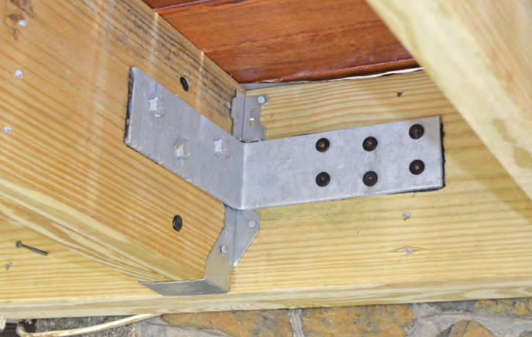
Figure 10. At the suggestion of his building inspector, the author rotated one of his custom L-brackets horizontally and fastened it to a solid 4-inch by 6-inch sill with HeadLOK screws. The bracket needed to be fastened to the doubled joist with three bolts instead of two, which required an additional hole drilled through the bracket.
