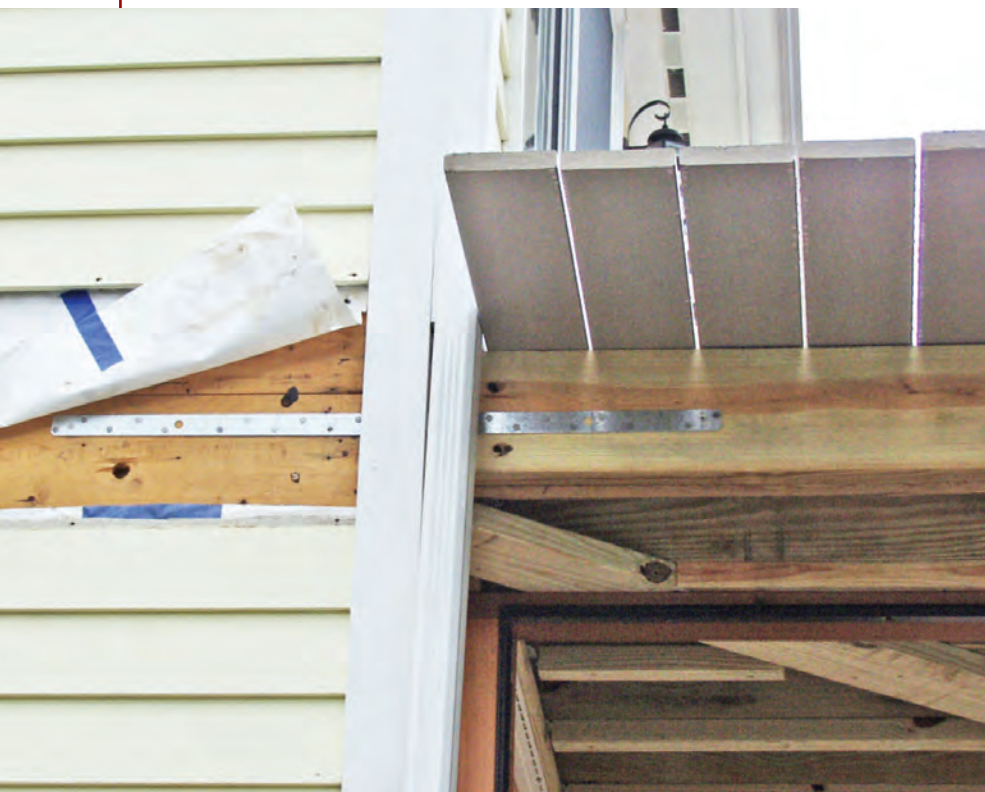
Figure 6. When the deck framing is aligned with the house framing, a simple metal strap can provide sufficient strength to meet lateral load requirements. On existing construction, the siding and sheathing must be temporarily removed to gain access to the framing.
