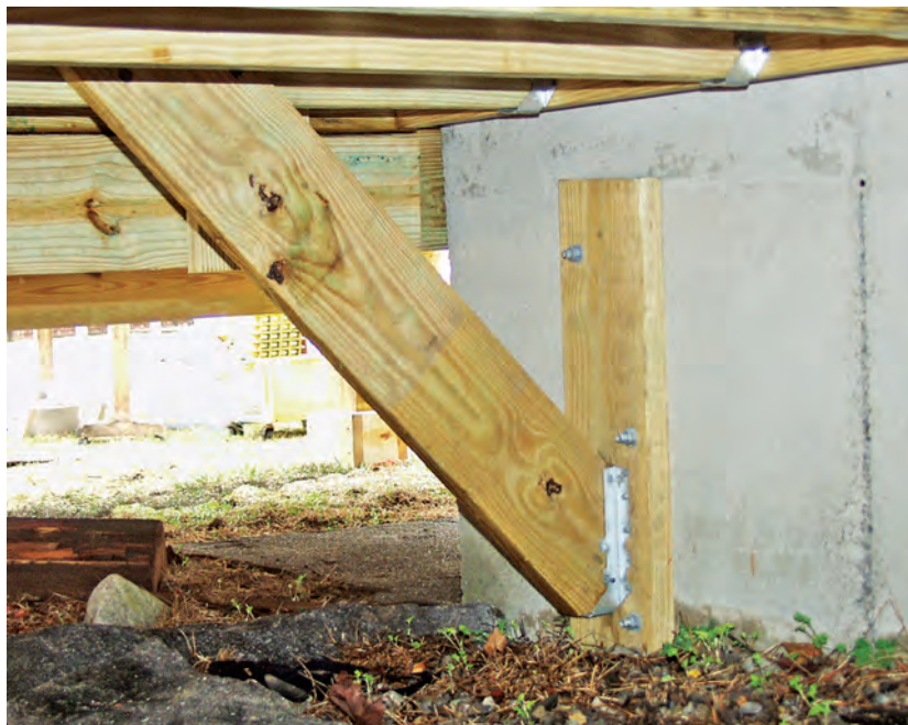
Figure 8. While this lateral load anchor hasn't been stamped by an engineer, it may be an option that would be approved by your building inspector. Here, a single 2x8 diagonal brace is through-bolted to a joist and fastened to the foundation with a joist hanger attached to blocking.
