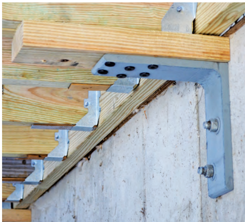
Figure 5. Sometimes blocking is required to avoid installing concrete anchors too close to a foundation edge. In those cases, the author uses 6-inch instead of 4½-inch-long HeadLOK screws to attach the bracket to the doubled joists. The bracket in the photo was fabricated from ½-inch-thick angle iron (the steel was manufactured as a 16-foot-long angle bar with two 8-inch flanges). While the steel is much thicker than necessary, it was readily available, and the fabricator could just cut off 3-inch-wide pieces of the angled steel.
