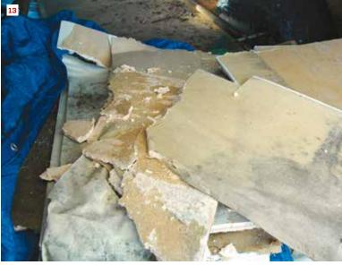
Air movers or carpet fans (12) create a high-volume stream of air to pull moisture from the surfaces of materials into the air; a dehumidifier condenses moisture from the air into water that can be carried out of the building. In moderate temperatures, water-soaked materials can easily develop mold before they are able to dry (13). Mold discovered during cleanup should treated—preferably by a mold remediation specialist and removed from the building.
