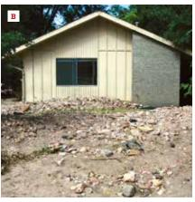
The sheer volume of debris quickly filled city-supplied roll-offs, prompting residents to dump debris on the ground nearby, blocking haulers' access (A). Sand and sediment near buildings (B) was assumed to be contaminated with chemicals and sewage, and had to be hauled to landfills rather than re-used as fill.
