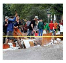
Sandbags slow but do not stop the flow of flood water; still they can prevent damage to finishes, appliances, and equipment caused by sediment and other particulates.
