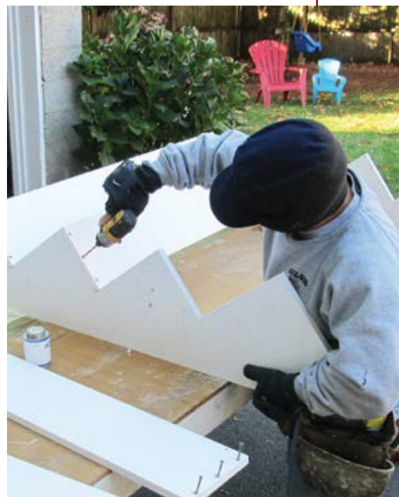
Figure 2. After ripping the PVC risers to size, the author fastened them to the notched skirtboards with PVC glue and countersunk coated deck screws.
