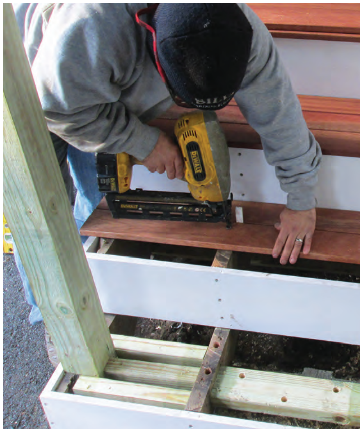
Figure 8. The pre-finished Meranti Batu treads were fastened to the stringers with 2-inch stainless steel finish nails, two nails per shim screw location.
