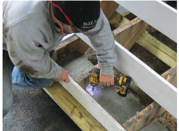
Figure 4. After the new concrete landing pad was poured, the middle stringers were trimmed to fit and attached to the pad with angle brackets.
