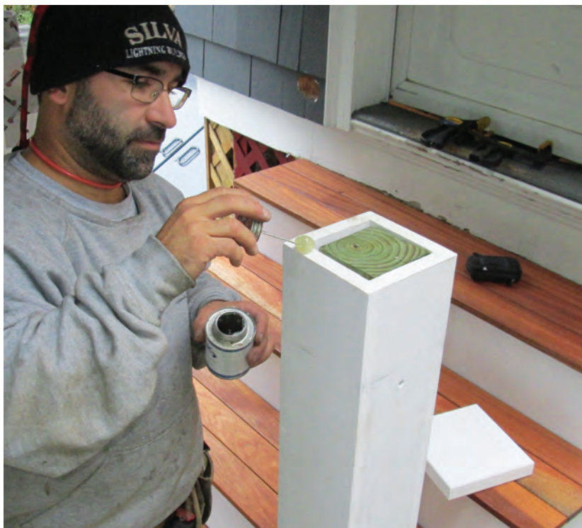
Figure 11. The post caps were made of a double layer of PVC, and were glued to the tops of the post wraps. The author used masking tape to hold the caps in place while the glue cured.
