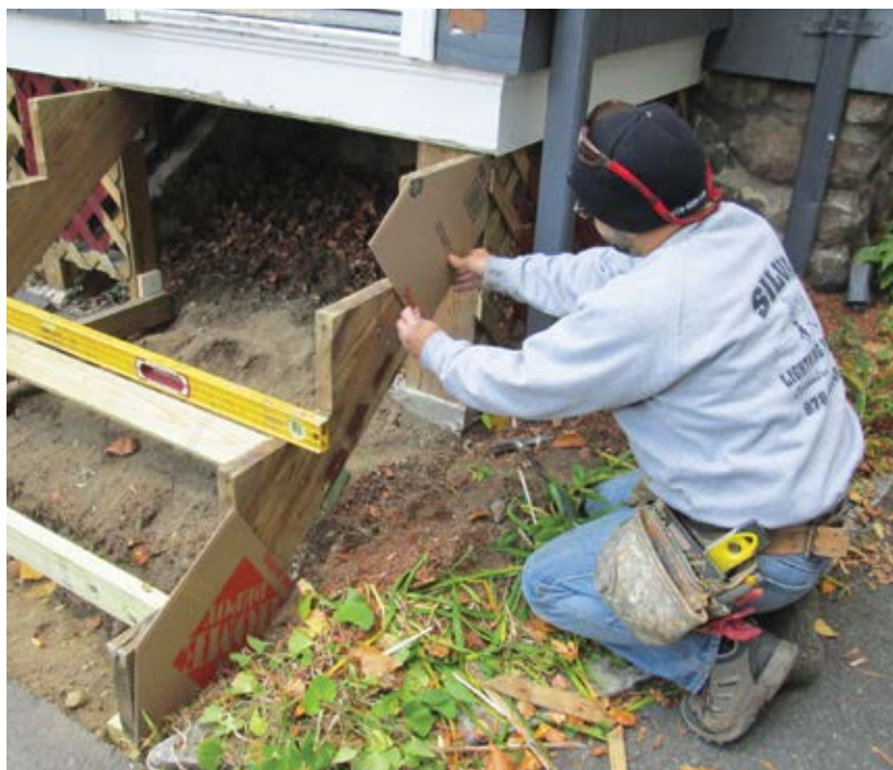
Figure 1. The author cut out two cardboard templates, one for each end of the stringer. Adding the distance between the templates to their lengths gave him the exact dimensions for the PVC skirtboards that would cover the stringers.
