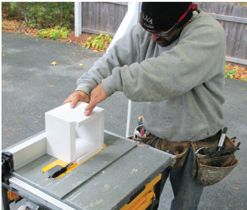
Figure 10. The author assembled the PVC post bases with glue and nails, then beveled the top edges at a 30° angle.
