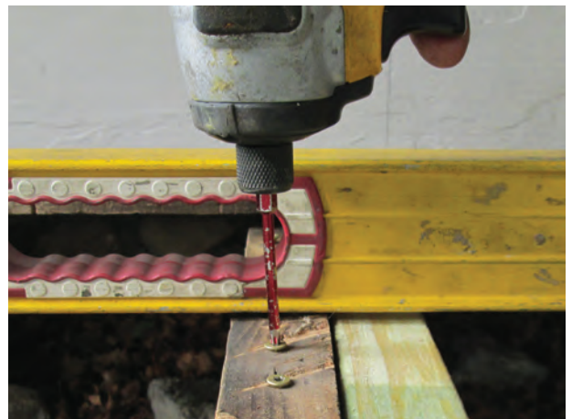
Figure 5. The author predrilled holes for the broad-headed shim screws that he would use to level the individual boards making up the treads. A simple jig helped ensure that each screw would be in the right location.
