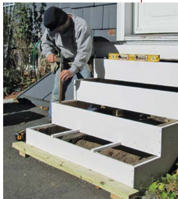
Figure 3. Shims were used to level and square up the PVC skirt-riser assembly before it was screwed to the stringers.
