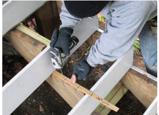
Figure 5. The author predrilled holes for the broad-headed shim screws that he would use to level the individual boards making up the treads. A simple jig helped ensure that each screw would be in the right location.
