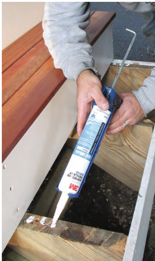
Figure 7. Before installing the hardwood treads, the author applied marine adhesive to the head of each shim screw.
