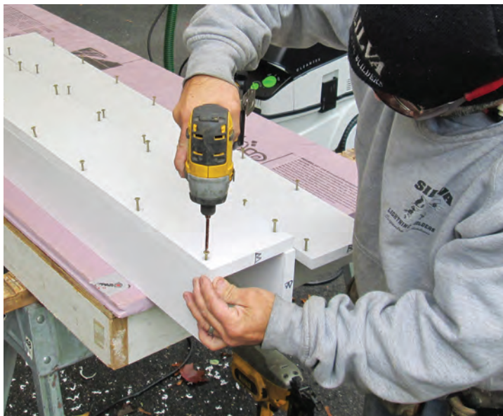
Figure 9. The PVC post wraps were fastened together with glue and countersunk screws spaced 6 inches apart.
