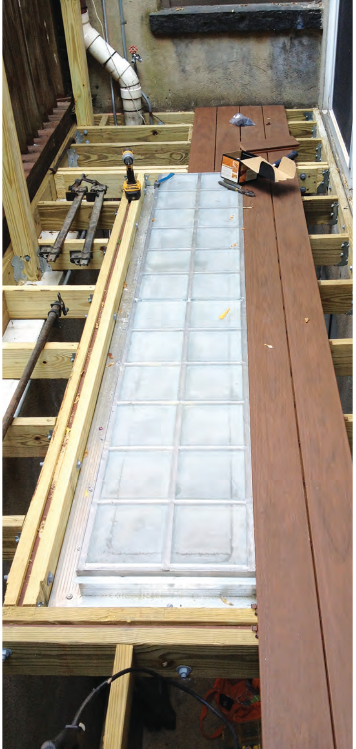
Figure 6. With the skylight secured to the framing, workers installed the TimberTech XLM decking, which was secured to the joists with hidden fasteners. The decking was laid out from the edge of the skylight rather than from one of the deck edges.
