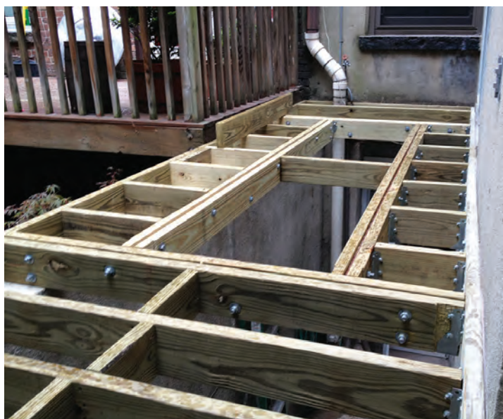
Figure 3. The deck framing is partially supported by a concrete-block separation wall. Doubled 2x6 joists used to frame the rough opening for the skylight were reinforced with 1/4-inch by 5-inch steel plates.
