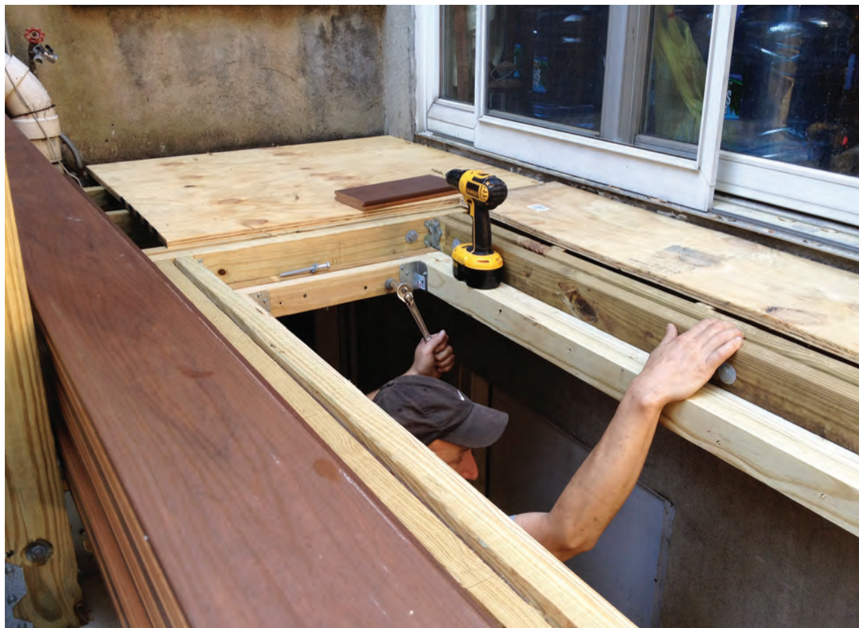
Figure 4. To support the skylight, workers glued, nailed, and bolted a 3-inch-wide ledge to the rough opening. Plywood was used as temporary decking during construction.
