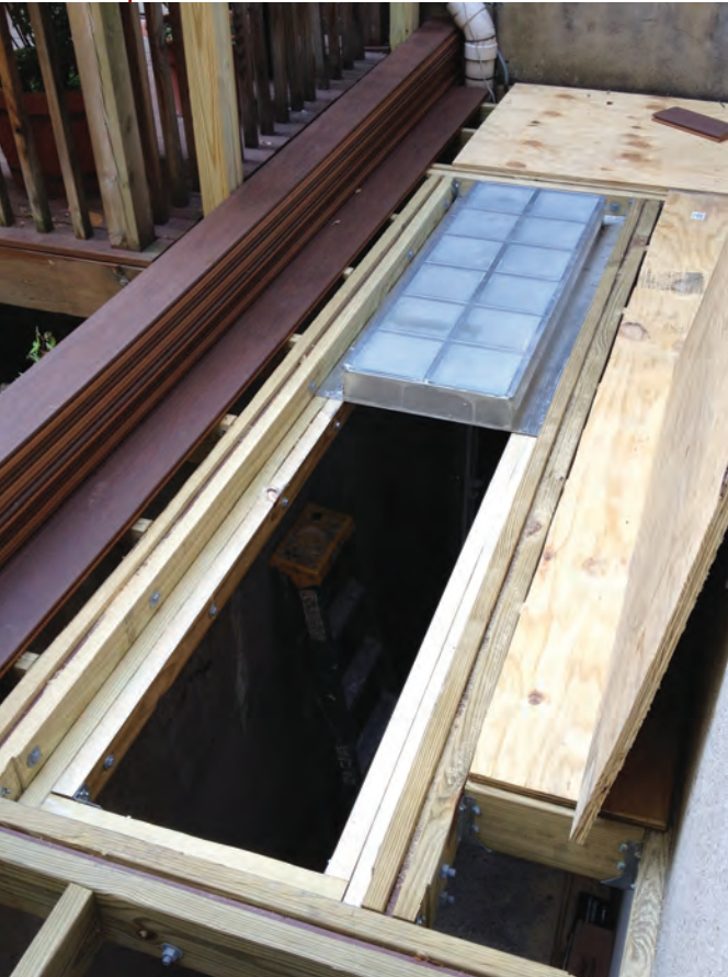
Figure 5. The skylight units were installed one at a time, with shims as necessary to level them and provide full bearing. Grey silicone sealant supplied by the manufacturer was used to fill the joint between the two units.
