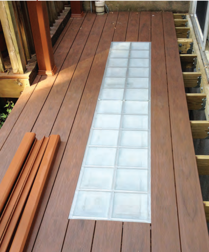
Figure 7. The skylight has a non-skid finish and is flush with the decking (above). TimberTech RadianceRail finishes the deck off (top right).
