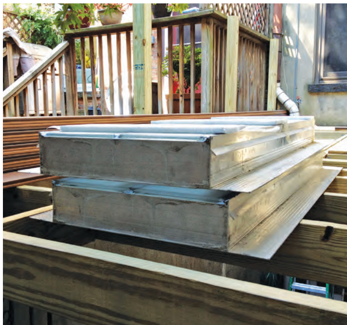
Figure 2. Structural glass-block skylights are heavy, so the author ordered two smaller units instead of one large one to make handling easier.
