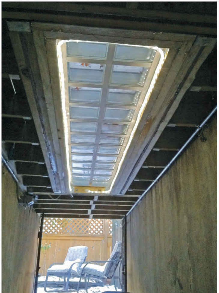
Figure 7. The skylight has a non-skid finish and is flush with the decking (above). TimberTech RadianceRail finishes the deck off (top right).
