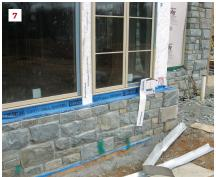
purpose-made plastic devices (although tubes tend to clog or become insect nests), or drainable mesh (visible at the bottom of the wall in photo 7).
