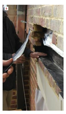
the seams simply lapped, not sealed. Water was draining off the housewrap and onto the head flashing, but it was leaking through the seams. Plus, there were no end dams, so water was spilling off each end of the flashing and finding its way past the housewrap, past a layer of foil-faced polyiso insulation, and into the wall (1).
